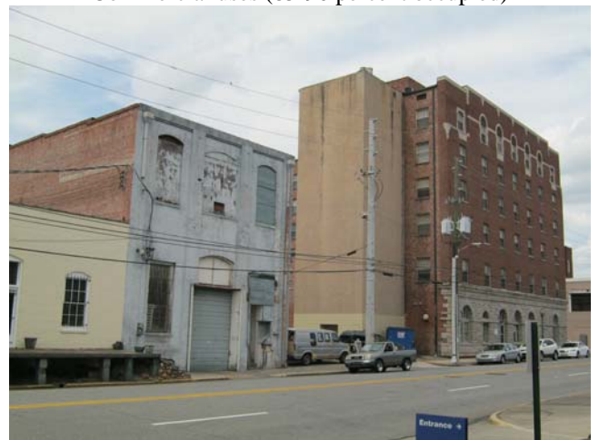
View of historic building adjacent to Subject
