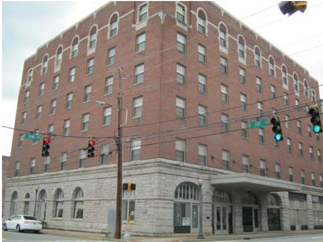
Subject (Portion with red brick exterior)
