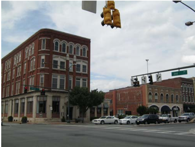
View of 2 nd Ave and Broad Street (Commercial corridor)
