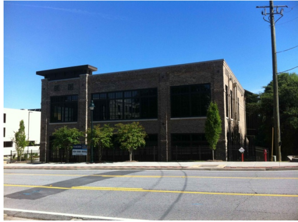
Integra Construction offices bordering site to the southeast
