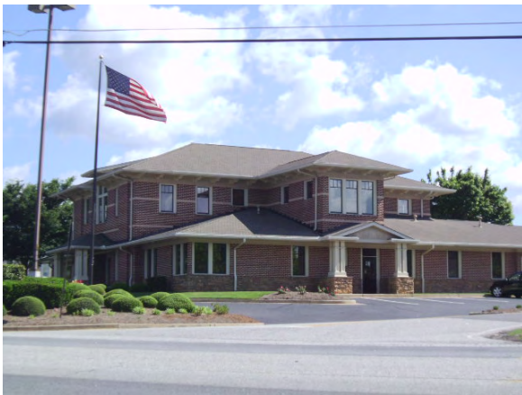
Public safety building, east of site
