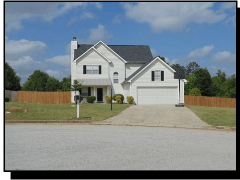
(4) Site located behind this dwelling w/in subdivision.
