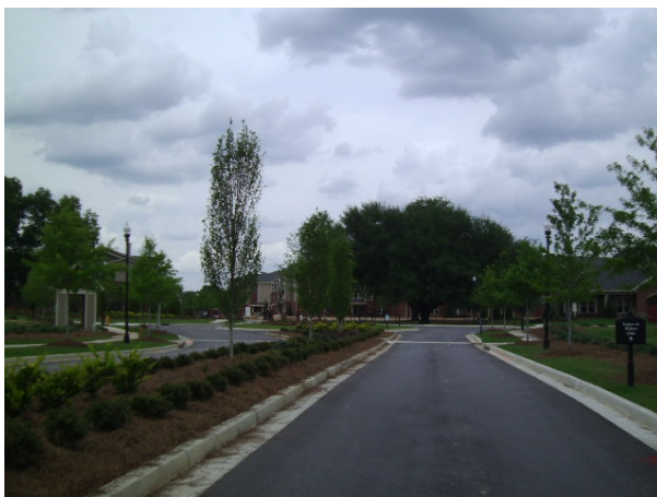
View of main entrance at Fairhope and Sand Bar Ferry
