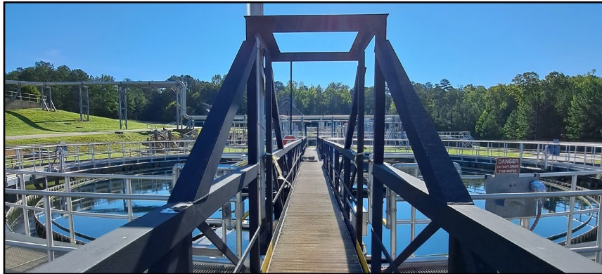
Figure 24. Cedar Creek Water Reclamation Facility in Athens-Clarke County
