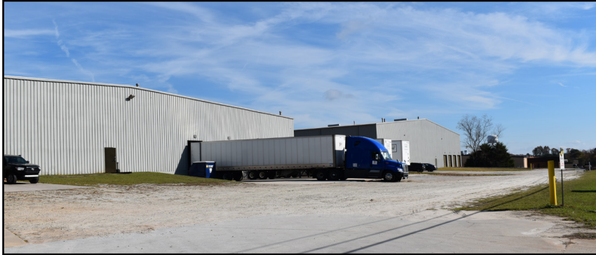
Figure 30. Industrial building along East Hightower Trail, east of downtown
