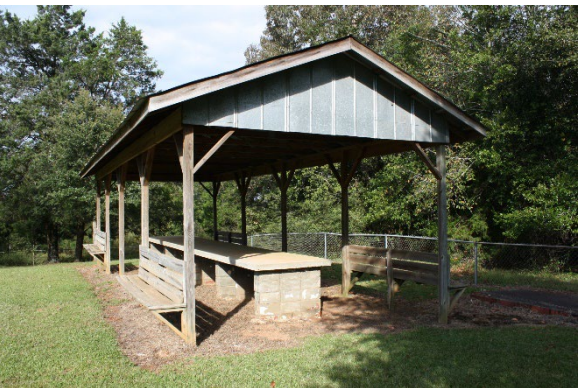
Photo 30: Northwesterly View toward open Pavilion
