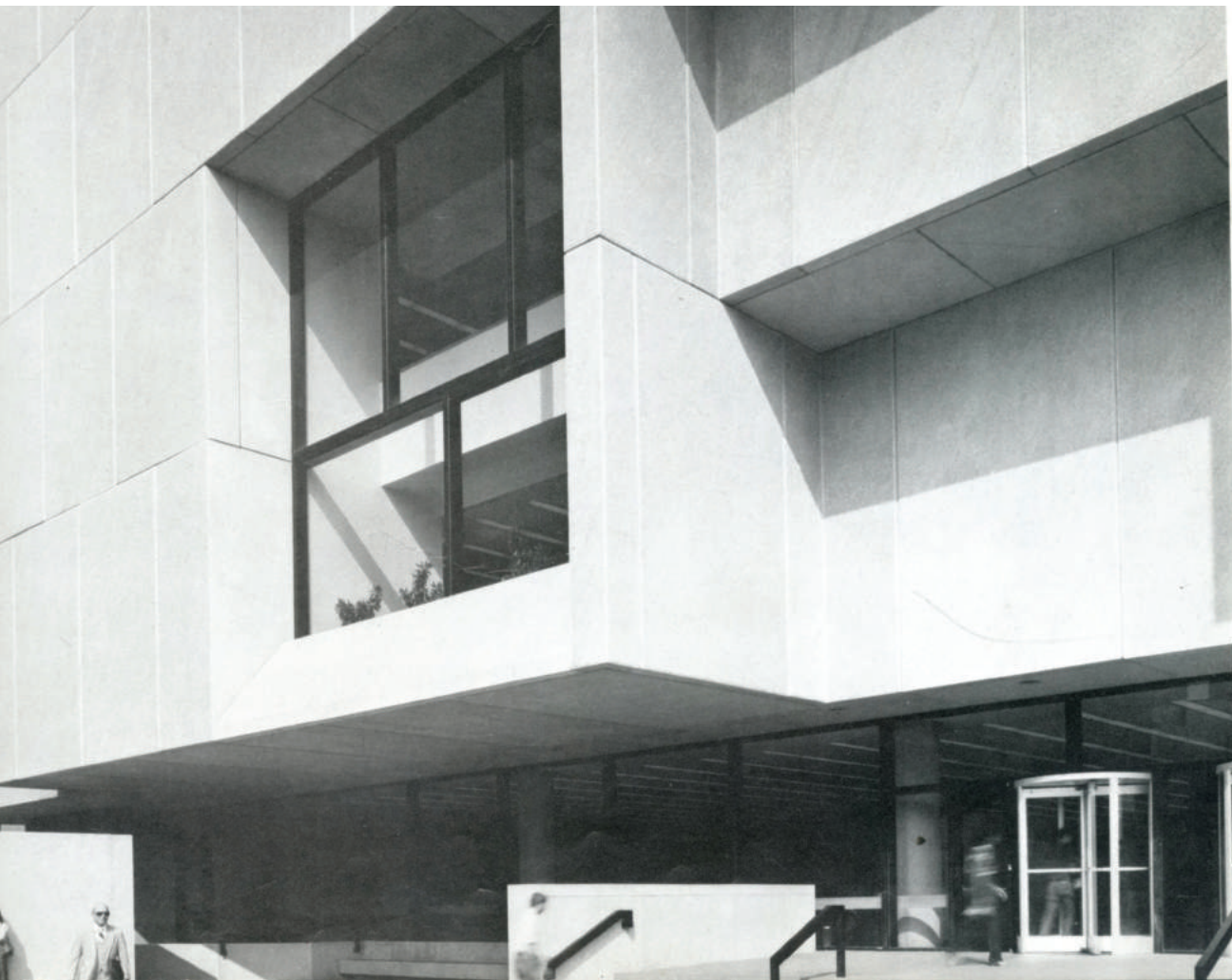
(Left) The Atlanta-Fulton County Central Public Library, 1981.
