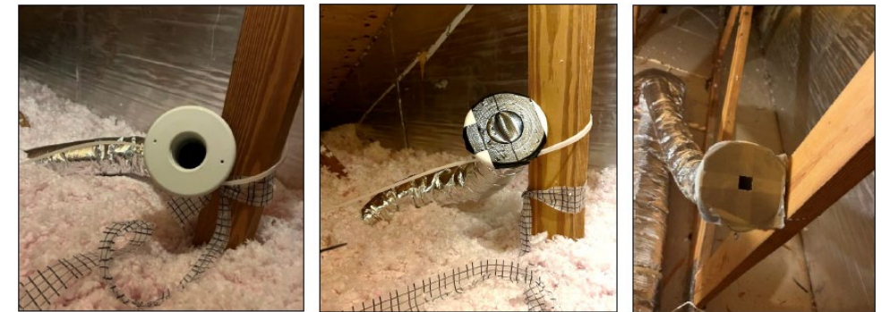
Smaller test attics required some engineering to get 50cfm/1000sf
