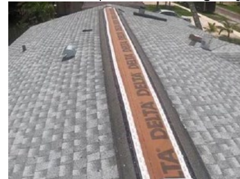
Vapor Diffusion Vent @ Ridge (prior to ridge vent installation)
