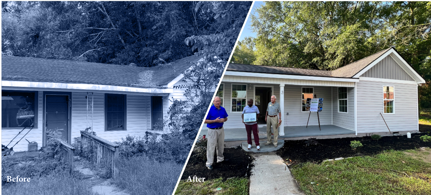
Dublin-Laurens County Land Bank Authority Housing Renovation Project
