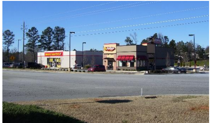
Commercial Development at Old Pendergrass Road and U.S. Highway 129
