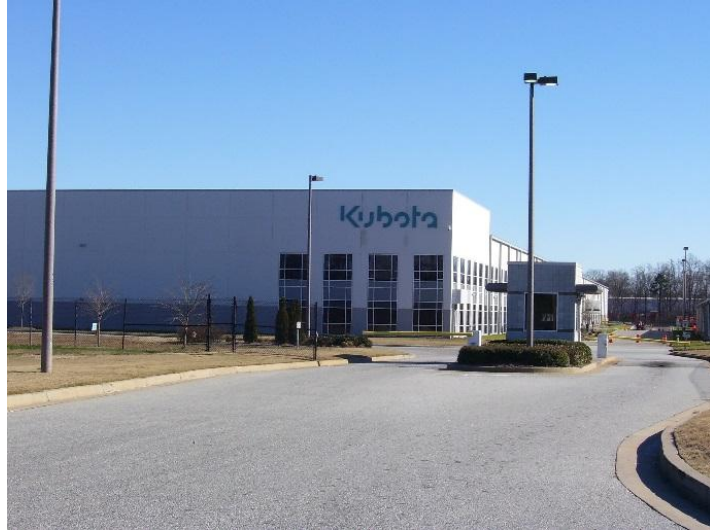
Kubota Building Addition
