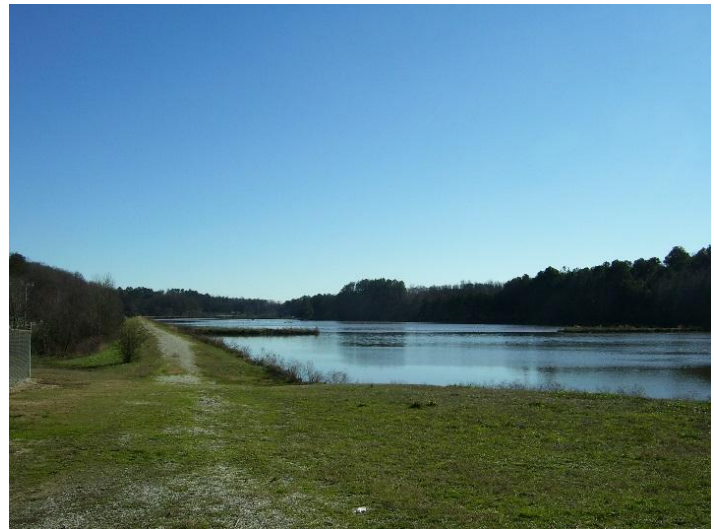
Curry Creek Reservoir
