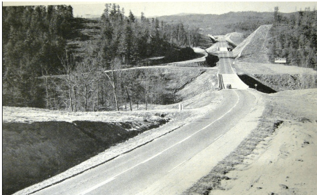
Figure 2. A factor in the ability to set higher geometric standards after WWII was the availability of larger, more powerful machines for grading and moving earthwork, allowing for economical construction of cuts and fills, as shown in this view of US 23/441 in Rabun County in 1960. In the 1920s and 1930s, this would have been too costly because of the heavy labor and time involved. Source: Biennial Report (1959-60).
