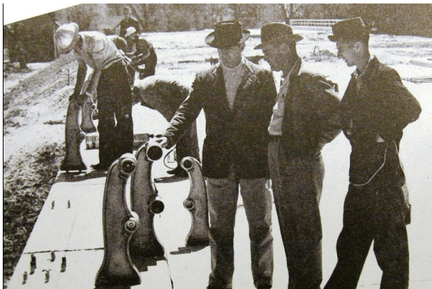
Figure 13. SHD engineers examine the standard aluminum railing posts for a bridge on the US 1 expressway in Augusta. Source: Georgia Highways (1958).
