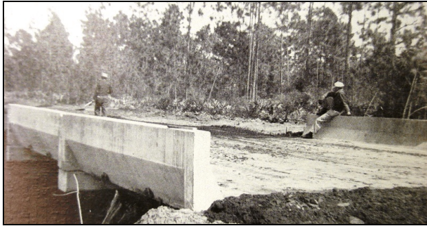
Figure 14. “Harry Brown” type, precast slab bridge. Source: Georgia Highway Proceedings (1957).
