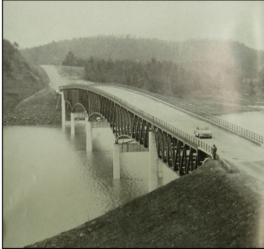
Figure 10. SR 53 over Lake Lanier, built in 1956. Source: Dixie Contractor (1956).
