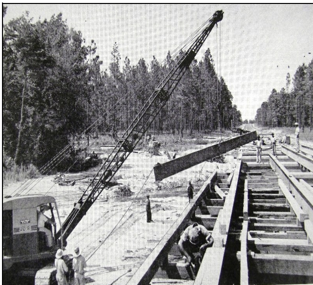
Figure 6. Erecting a steel stringer bridge near Albany. Source: Dixie Contractor (1960).
