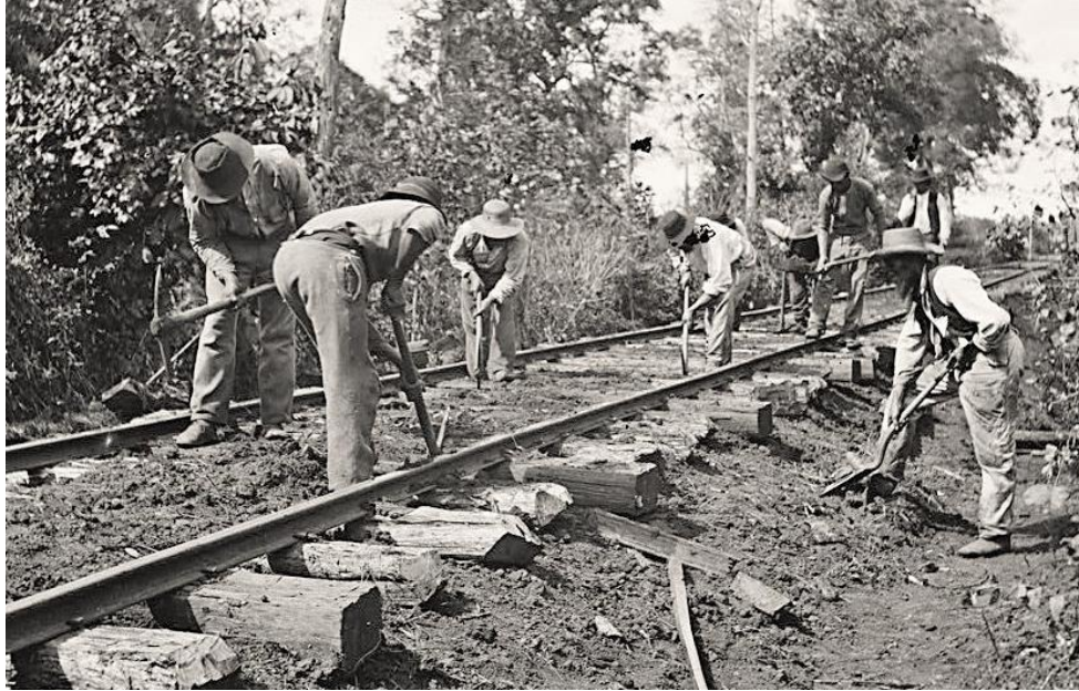
Figure 7. African Americans building a railroad in South Georgia in 1859 (Georgia Archives).
