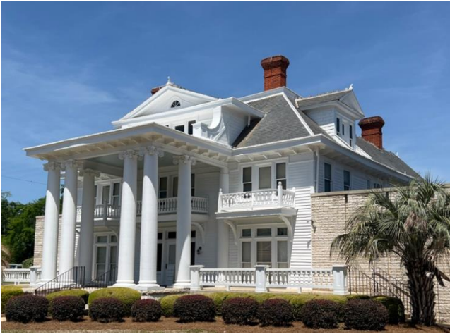
Figure 26. Example of Neoclassical Revival style building, No. 54804.
