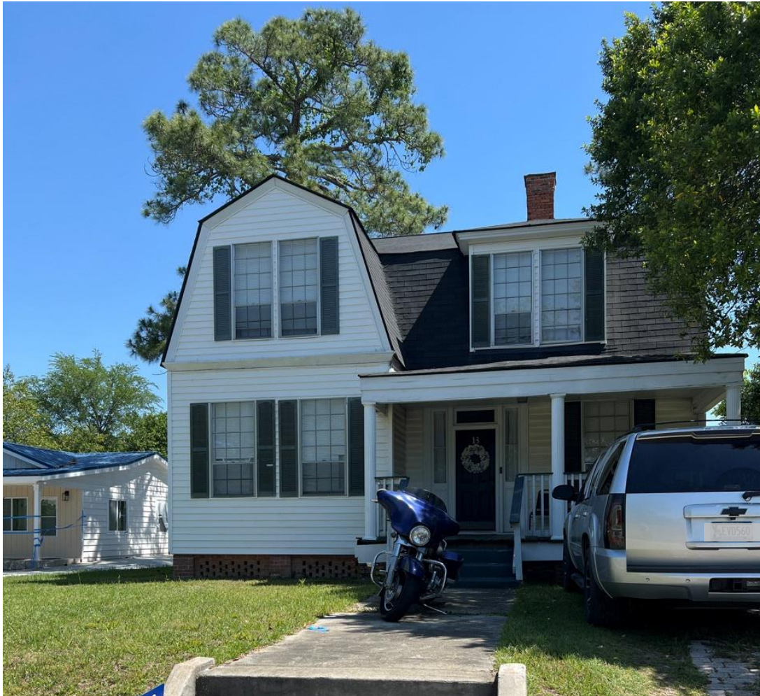
Figure 20. Example of a Dutch Colonial Revival in Hawkinsville, No. 287232
