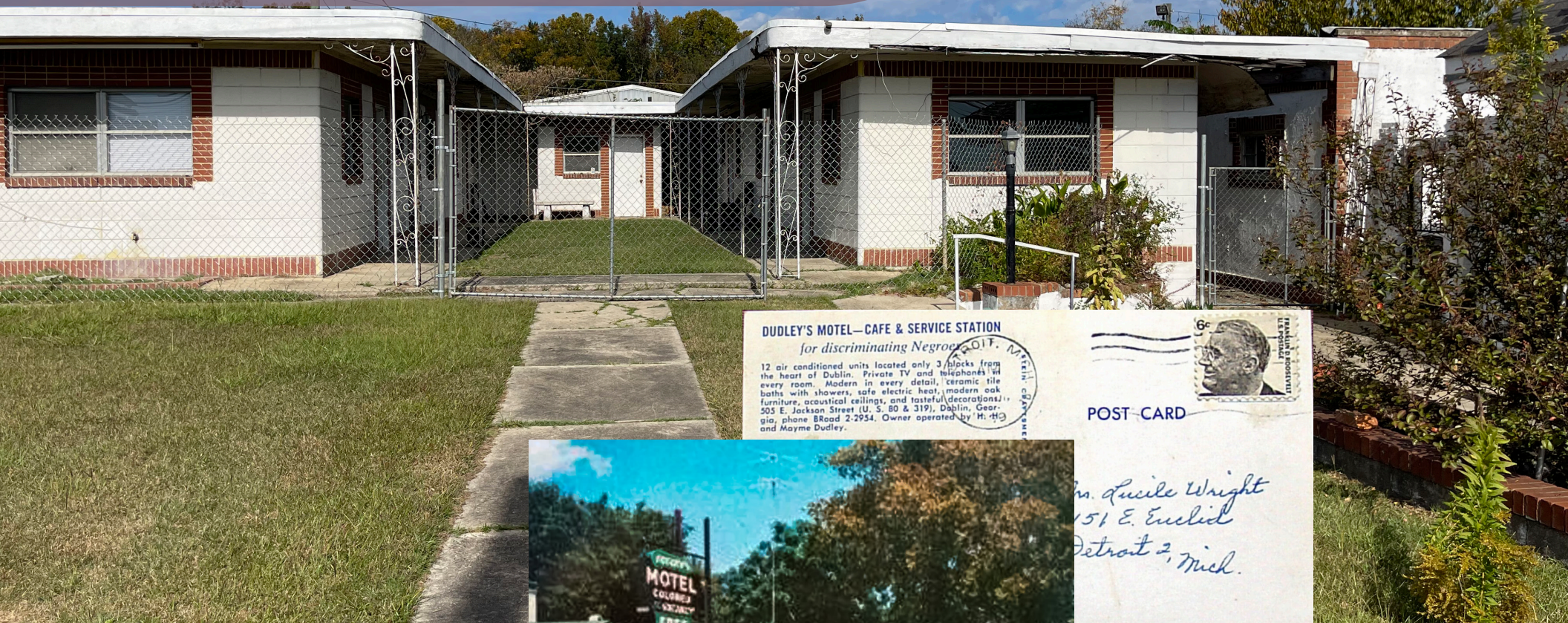
Dudley Motel (extant) in Dublin, Laurens County, called “One of the finest and most modern Negro motels to be found anywhere in the nation” when it opened in 1958. Courtesy of the Georgia Trust for Historic Preservation.
