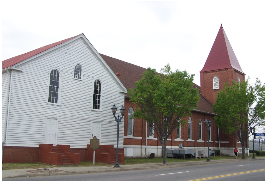
Springfield Baptist Church (extant) (NRIS #82002461) at 114 12th Street in Augusta, Richmond County, 2008. J. Stephen Conn.
