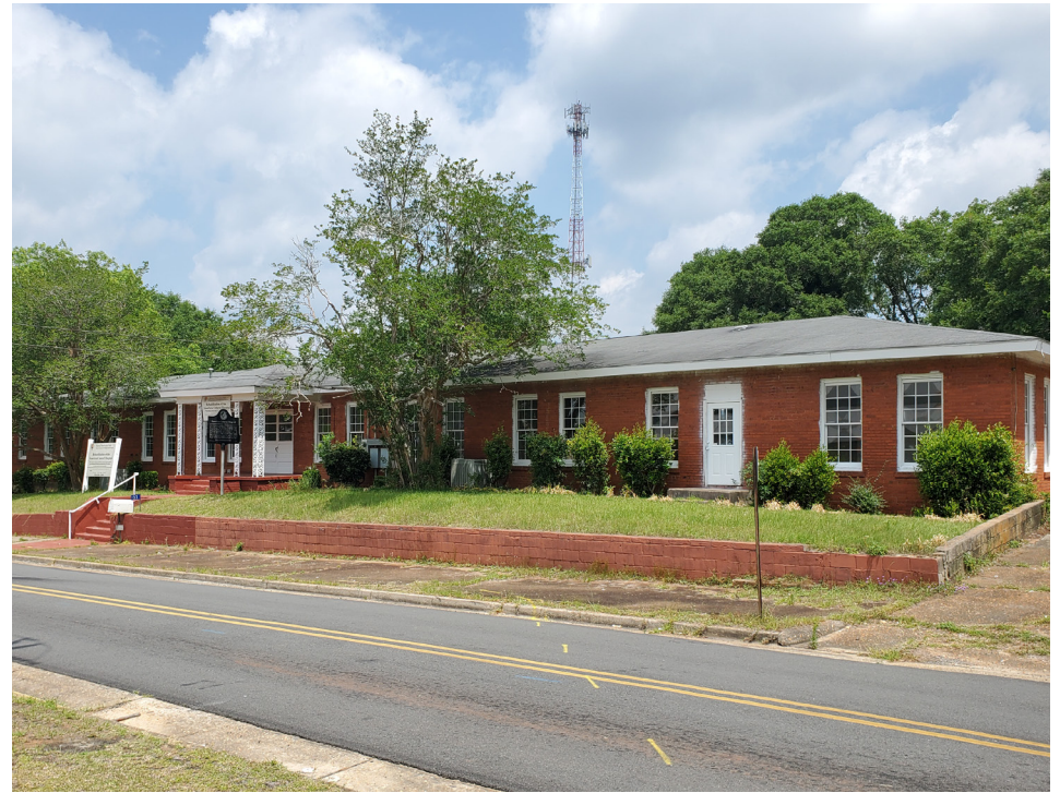
Americus Colored Hospital, 133 J.R. Campbell Sr. Street, Americus, Sumter County. One of the earliest hospitals for African Americans in southwest Georgia, constructed in 1923, which later served as the site of a Freedom School. Brandy Morrison.
