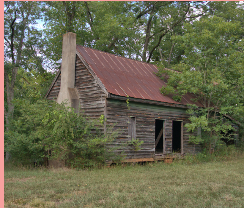
Boswell Tenant Housing at 1464 US-129, Eatonton, Putnam County. Built in the early 1800s as a Double-Pen with a side gable roof. A small family cemetery also exists on the lot. This resource is included in the National Register Nomination as an outbuilding to the Historic Tompkins Inn (NRIS #78001002). Brian Brown, 2022 .
