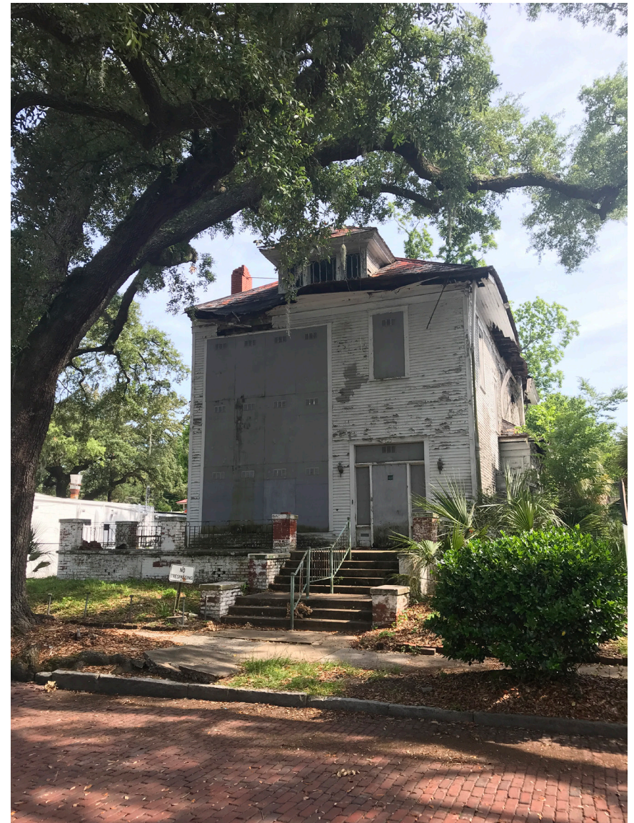
Kiah Museum (listing pending), 505 W 36th Street, Savannah, Chatham County. Ethos Preservation.
