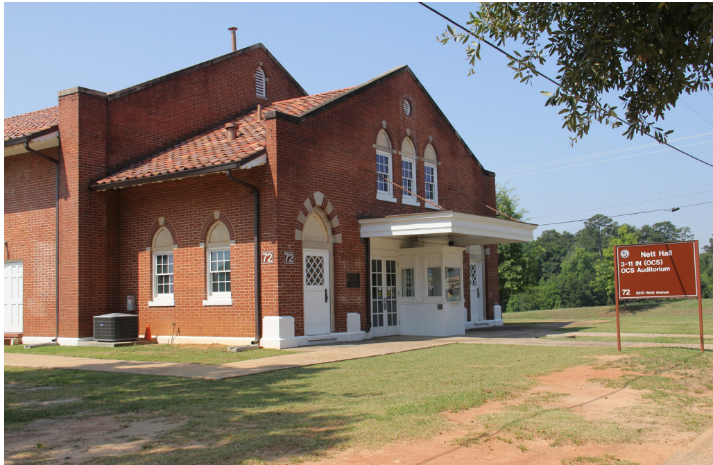
Nett Hall [extant], Fort Moore [formerly Fort Benning], Columbus, Muscogee County. U.S. Army photo by Edward Howard, U.S. Army Garrison Fort Benning Directorate of Public Works.
