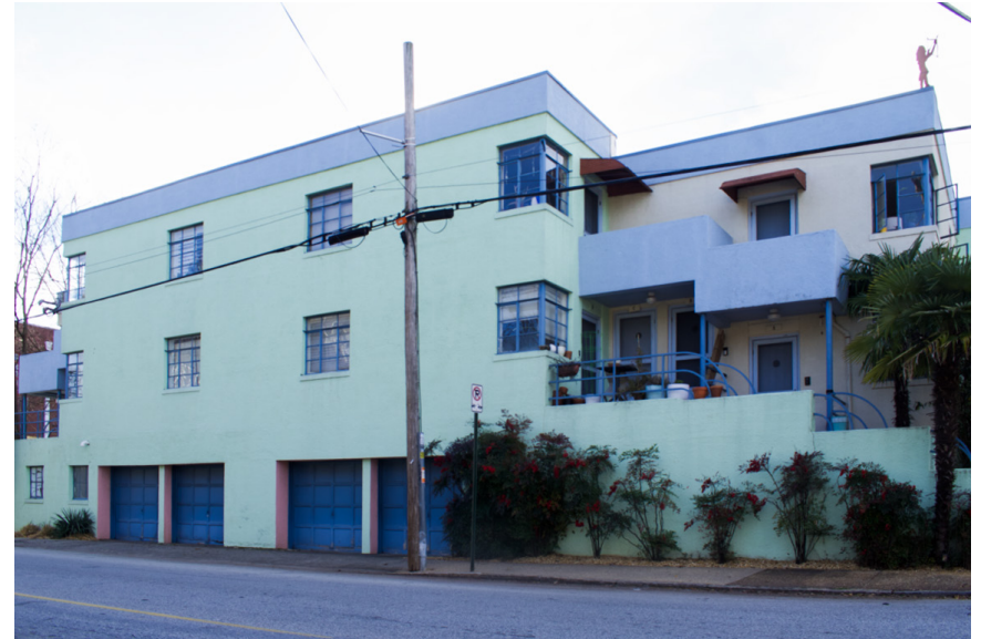
Wigwam Apartment Complex (extant) at 589 Auburn Avenue NE in Atlanta, Fulton County, built by Cornelius King and Sons. 440 Nedra Deadwyler.
