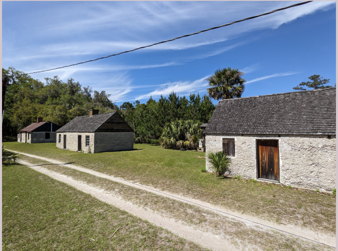
Slave Dwellings on Ossabaw Island (NRIS #96000468), Chatham County (extant). Ethos Preservation .
