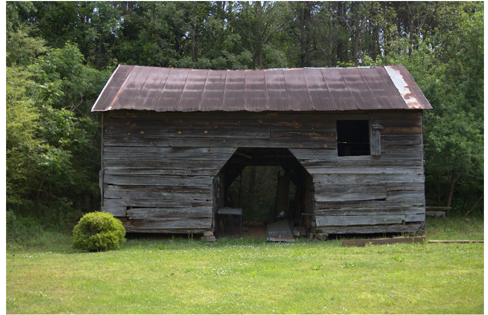
Double Crib barn on the c.1917 T. A. Bryant Homestead at 3956 Crossvale Road in Stonecrest, Dekalb County (extant). Brian Brown, 2022.
