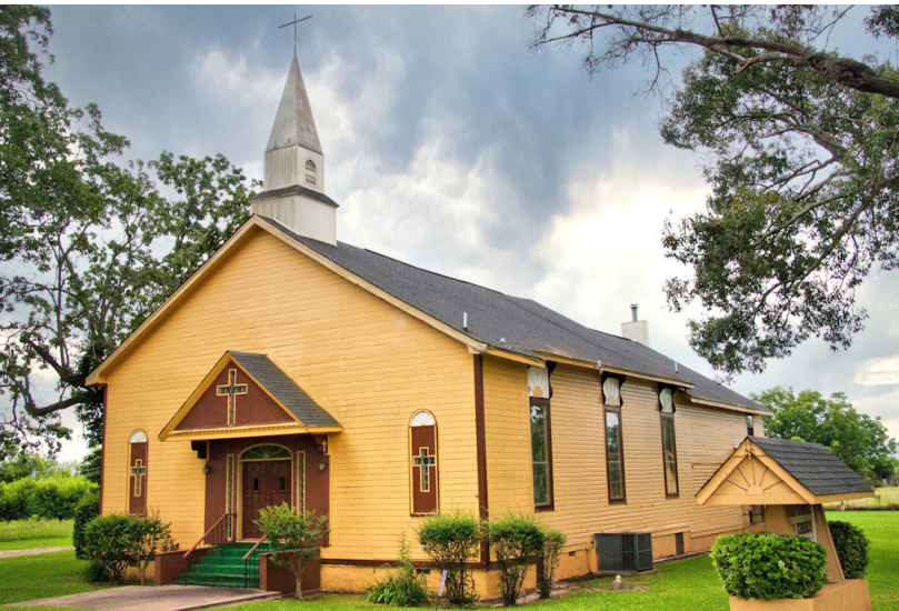
Front Gable Church, Allen Chapel AME Church at 9830 Miami Valley Road in Fort Valley, Peach County (extant). Brian Brown, 2023.
