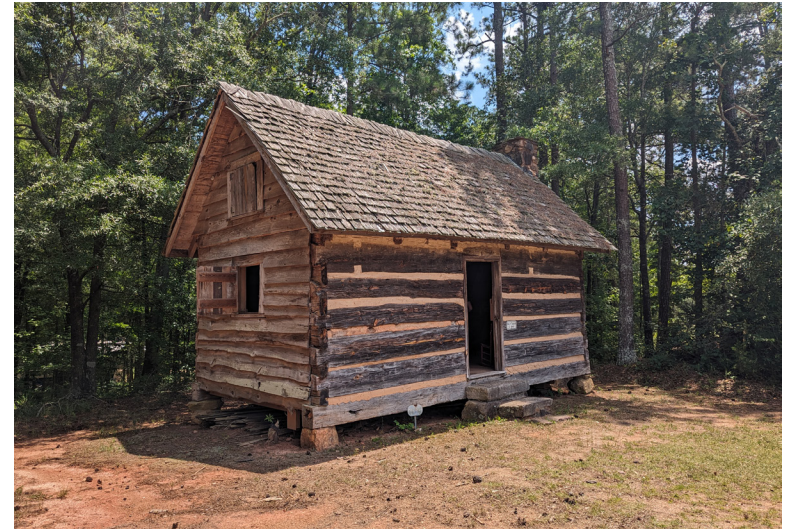
c. 1840 Double Pen Slave Dwelling (extant), moved from a plantation labor site operated by John William Dally in Walton County to the Arnold-Callaway Plantation (NRIS #72000402), 2160 Lexington Road, Washington, Wilkes County. Ethos Preservation .
