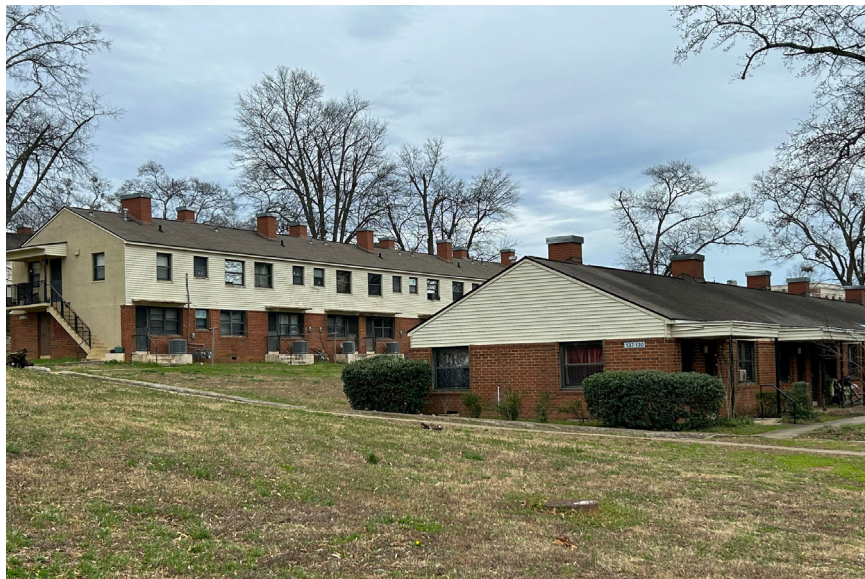
Parkview Homes (extant) off of South Newton Street north of Waddell Street in Athens, Clarke County. Bob Thomson.
