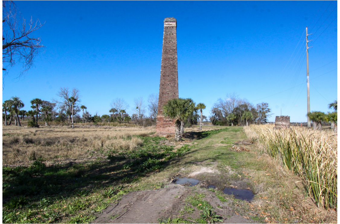
Butler Island Plantation labor site on Highway 17 south of the Darien River in McIntosh County. Ethos Preservation.
