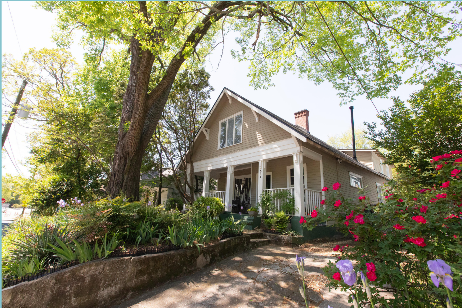
Artist Mildred Thompson’s home and studio [extant] at 361 Cherokee Avenue SE, a contributing resource to the Grant Park Historic District (NRIS #79000722) in Atlanta, Fulton County. Amanda Greene.
