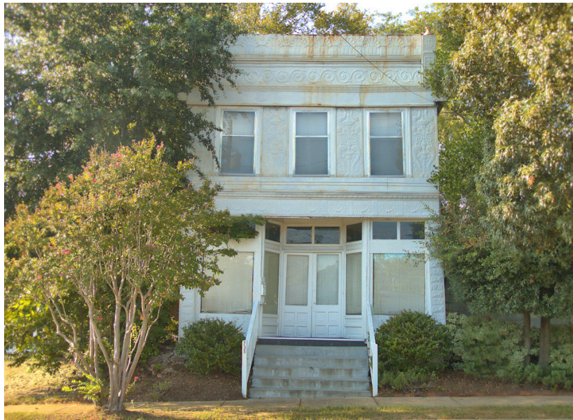
Toomer Building (extant) at 735 Carroll Street, Perry, Houston County, built in 1905. Brian Brown, 2023.
