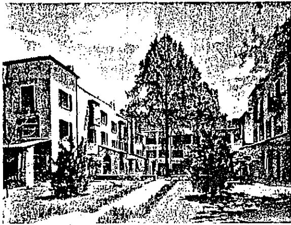
VIEW OF COURT
