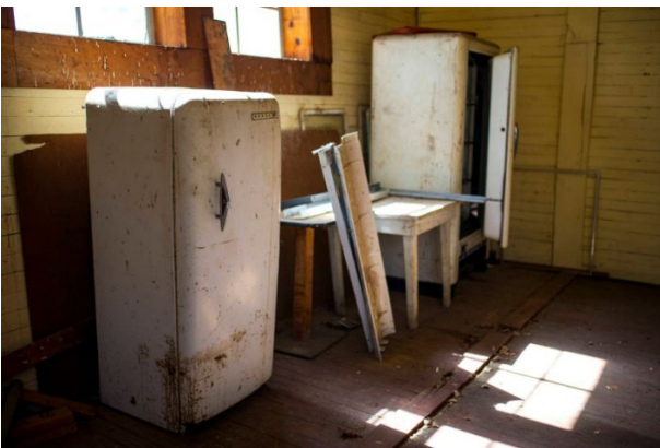
An interior image of the Springfield Log Cabin School and Community Center. Photo taken by Halston Pitman and Nick Woolever courtesy of the Georgia Trust for Historic Preservation
