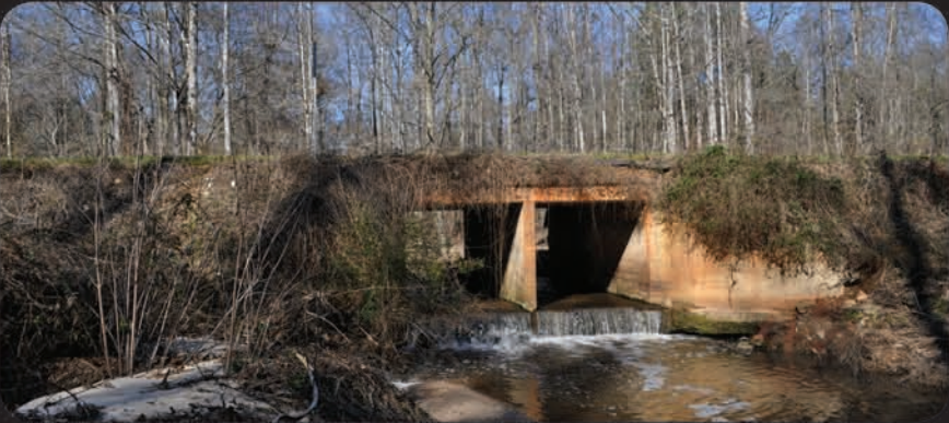
Cole Creek Culvert, Constructed 1939 , Lamar County
