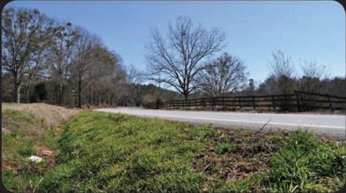
View of Dixie Highway
