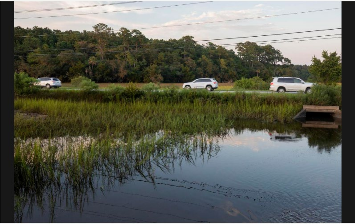
Figure 2.11 US Highway 41 crosses Horlbeck Creek in Mount Pleasant, SC. From the Post and Courier. https://www.postandcourier.com/news/charleston-county-offers-new-highway-41-plan-after-phillips-community-threatened/article_7e43f24c-7d21-11eb-9c93-ab7f799ffae1.html
