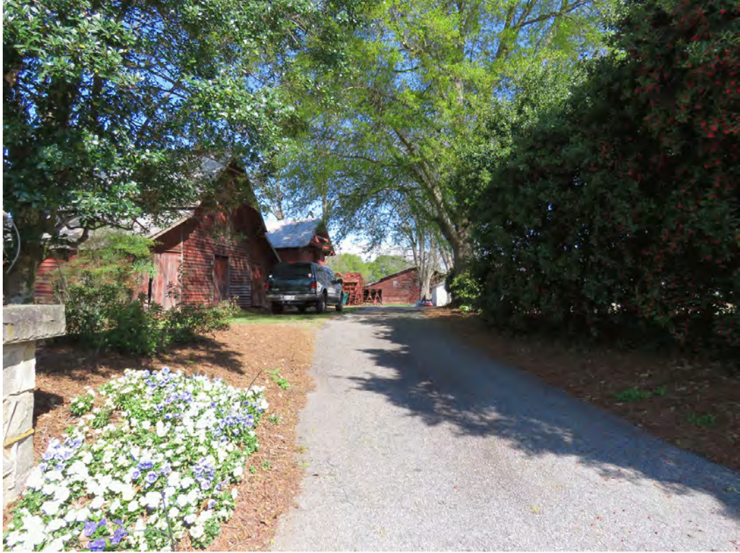
Photo 17 - View Looking North to Resource No. 28
