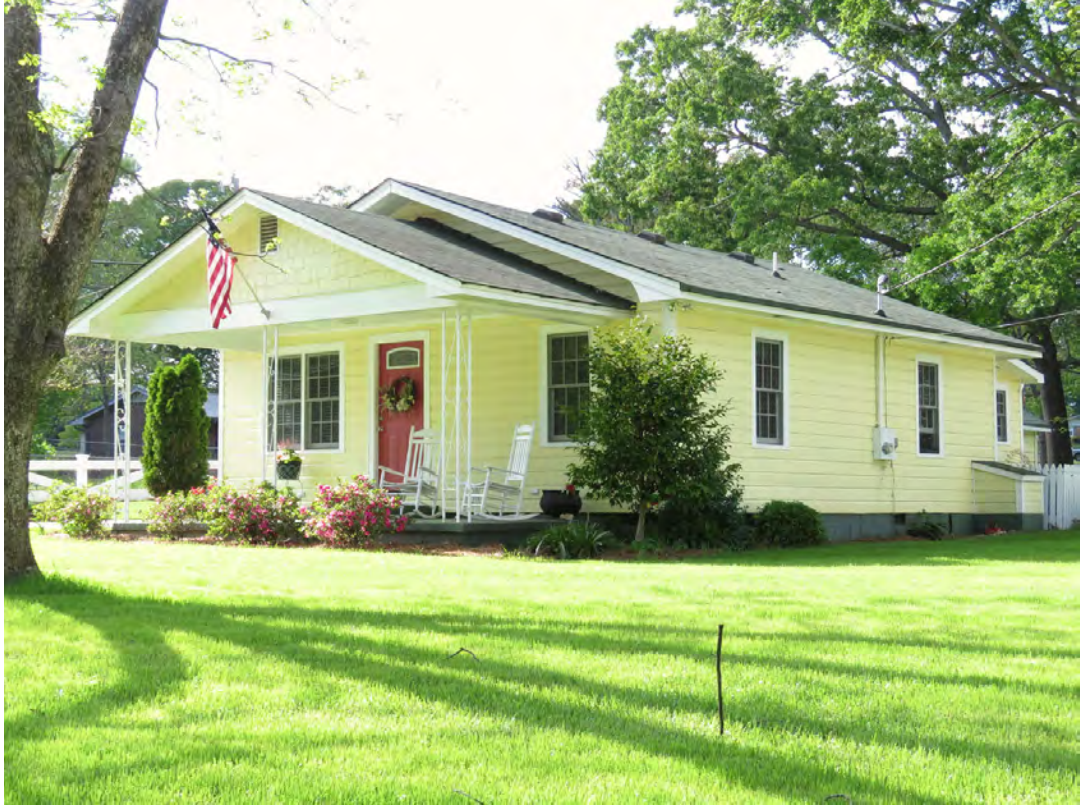
Photo 39 - View Looking Northwest to No. 55
