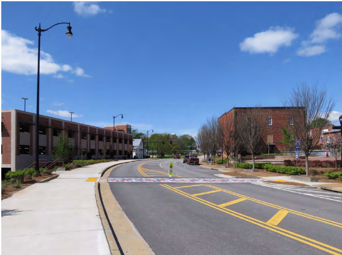
Photo 30 - Contextual View Looking Southwest Along Former Wall Street
