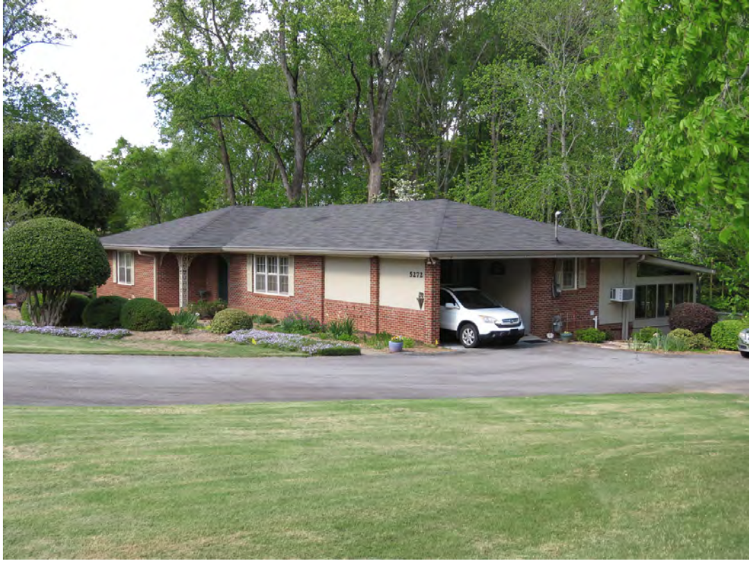
Photo 45 - View Looking Northeast to Resource No. 32
