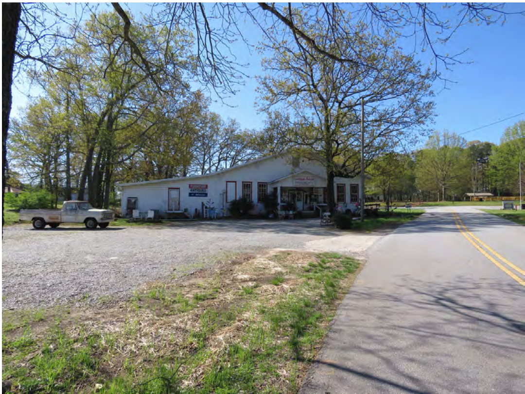
Photo 8 - View Looking Southeast to Resource No. 16
