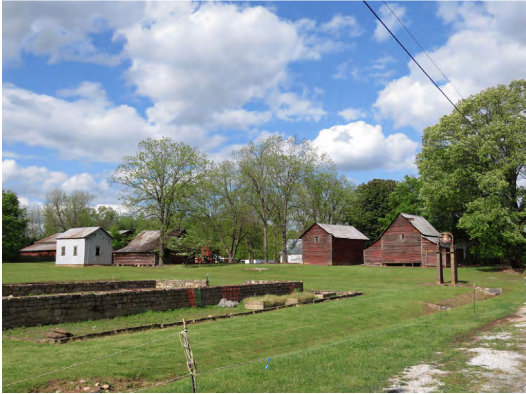
Photo 49 - View Looking Northeast to John Braselton Farm (Resource Nos. 26 and 28)
