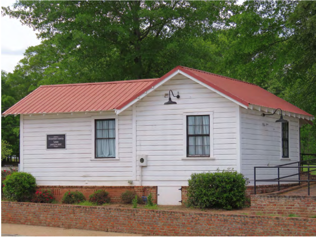
Photo 47 - View Looking Northwest to Relocated Resource No. 48/64
