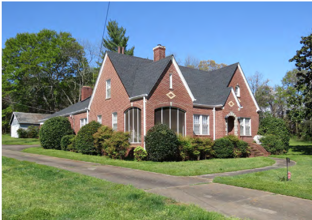
Photo 22 - View Looking Northwest to Resource No. 30
