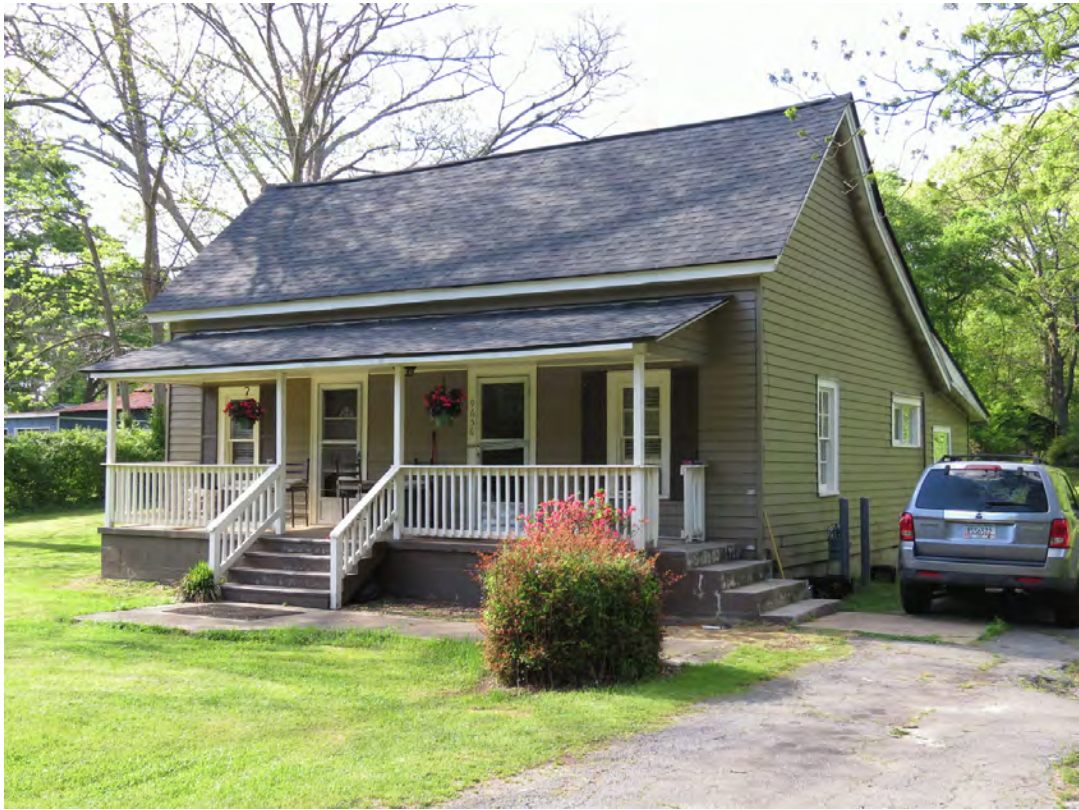
Photo 35 - View Looking Northwest to No. 57
