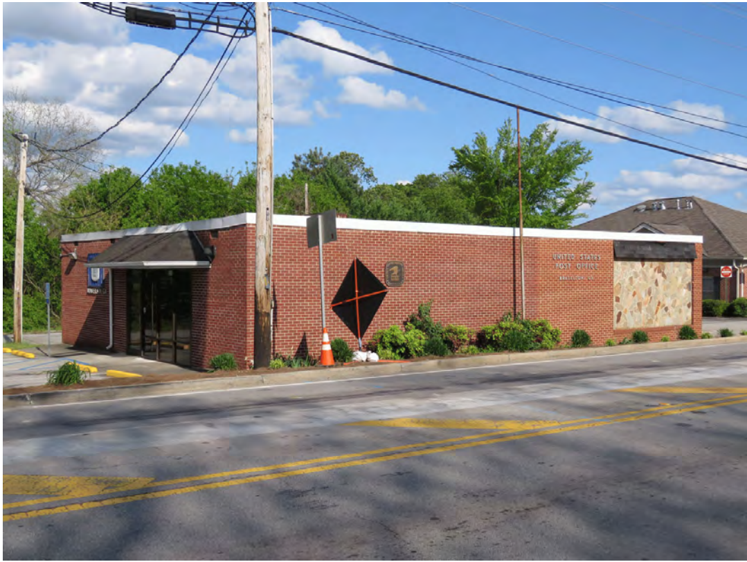
Photo 69 - View Looking Southeast to No. 33 (Post Office Building)
