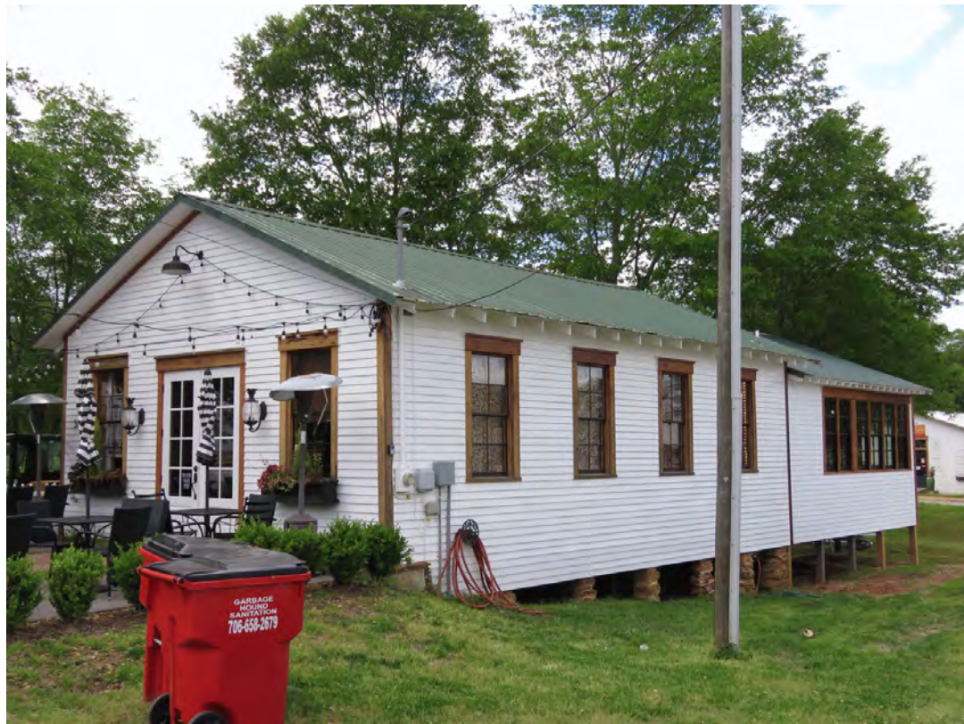
Photo 50 - View Looking Northwest to Resource No. 62
