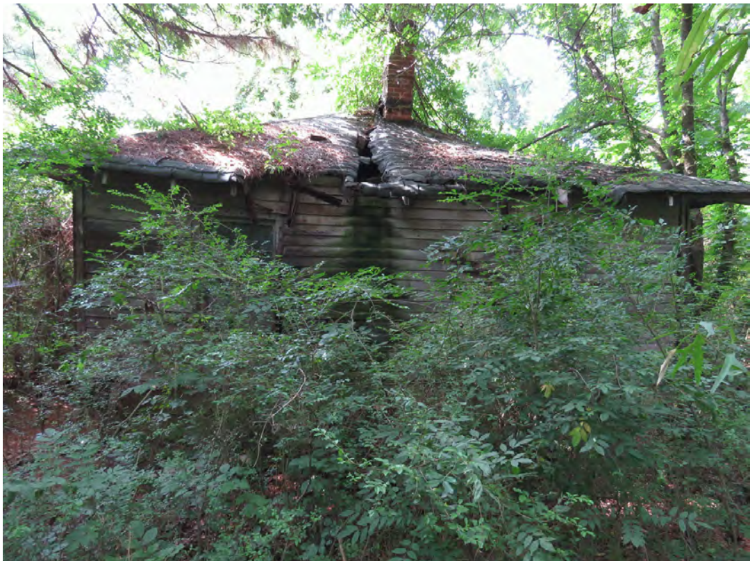
Photo 42 - View Looking South to Resource No. 35, North Side
