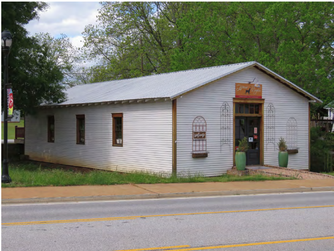
Photo 48 - View Looking Northeast to Resource No. 61
