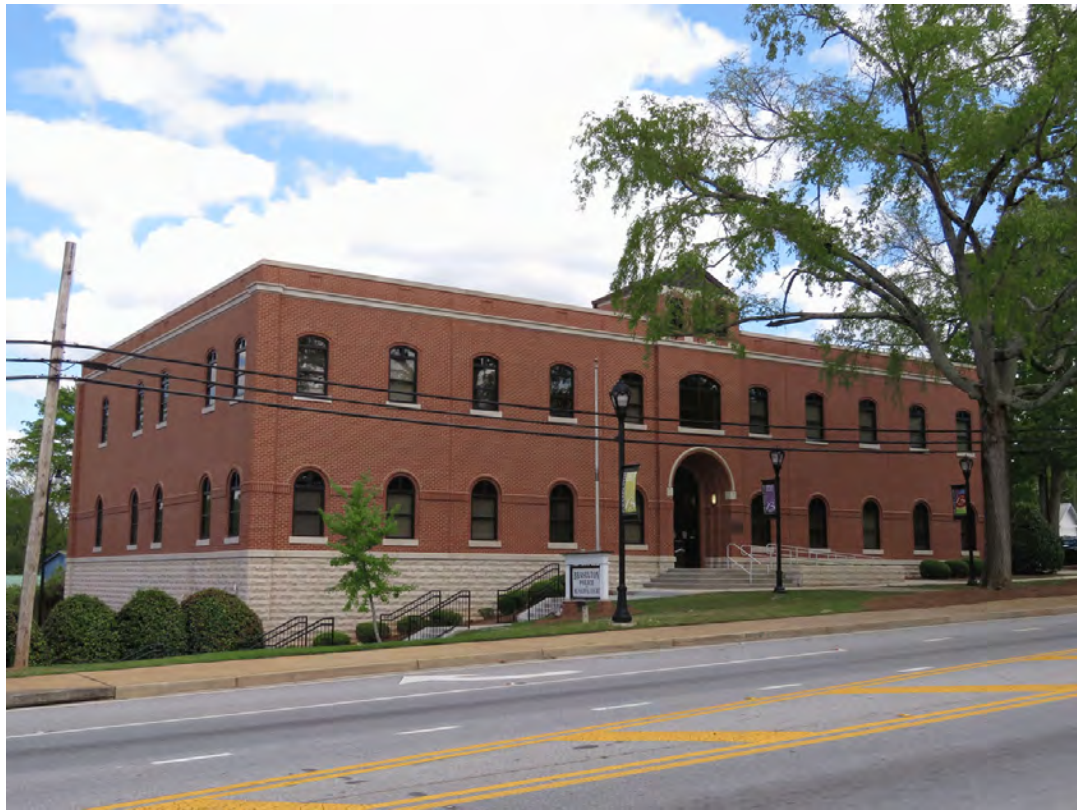
Photo 66 - View Looking Southeast to Modern Municipal Building, Site of Resource No. 20
