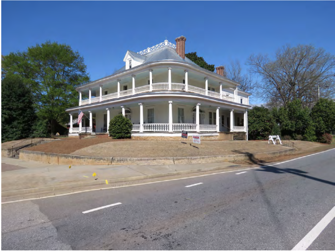
Photo 15 - View Looking West to the John Braselton House (No. 27)
