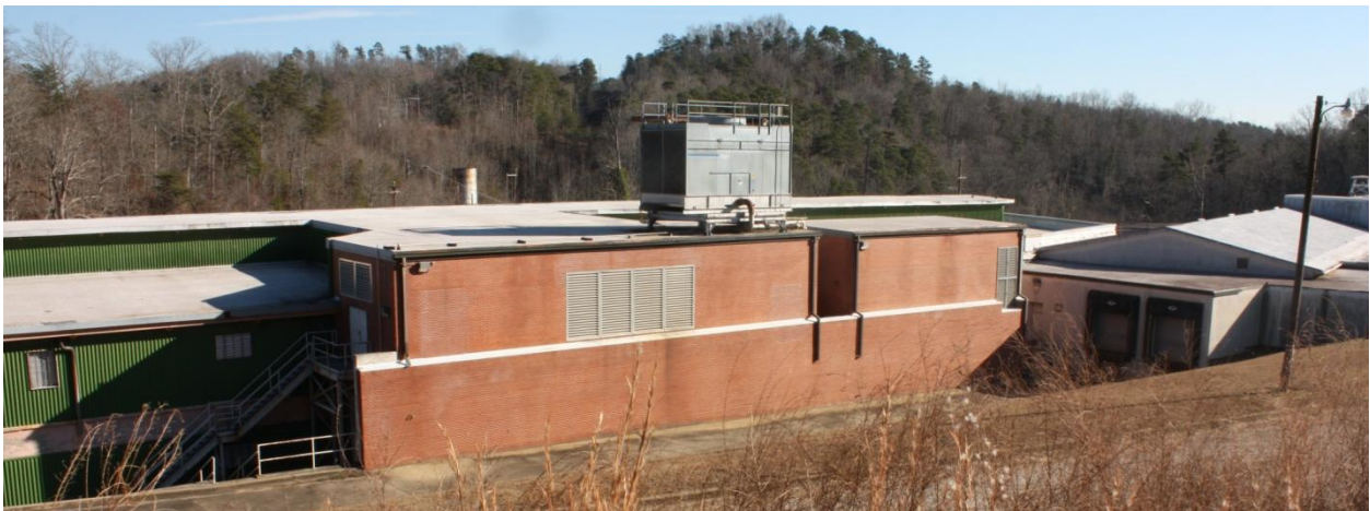
Figure 15: Photograph of Habersham Mills in Habersham County, Georgia. Photographer facing east, Photograph in possession of author taken December 9, 2010. Photograph of red brick addition added to house air washing and cooling system. To the left of the red brick addition, is the main mill which has been covered with corrugated metal.
