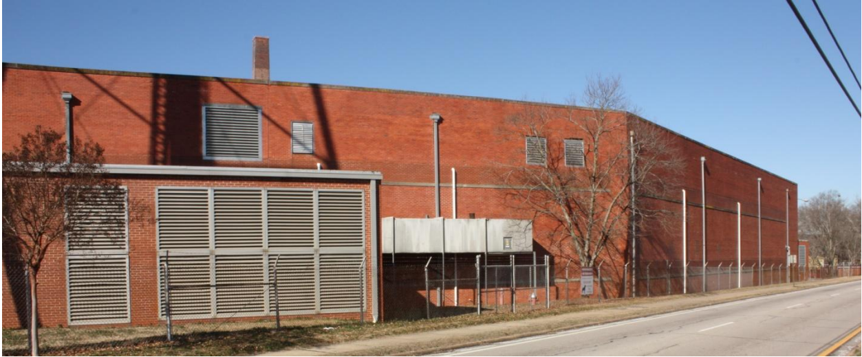
Figure 24: Photographer facing west, Photograph of multi storied windowless addition at Commerce's Harmony Grove Cotton Mills. Commerce, Jackson County Georgia, Photograph in possession of author taken February 8, 2011.
