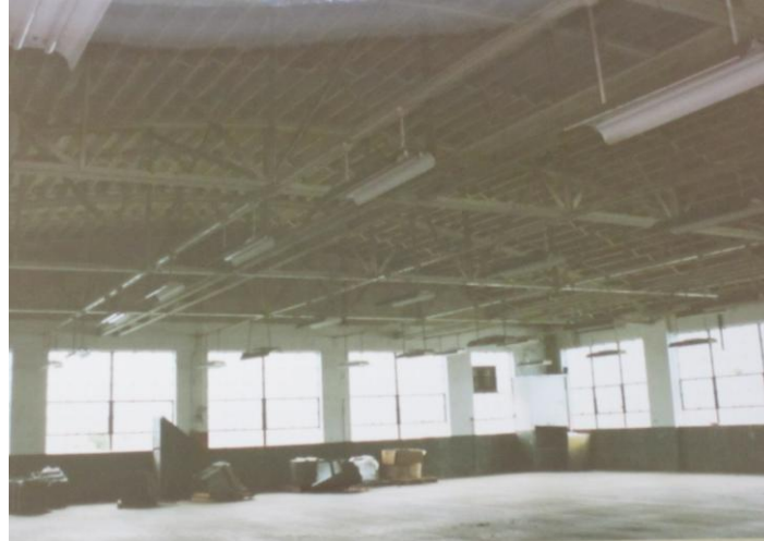
Figure 30: Photograph of Second of second floor interior, Building #5(1955 Addition) at Puritan Cordage Mills, Clarke County, Georgia, Photograph taken June 25, 1995 on file at Georgia Historic Preservation Division
