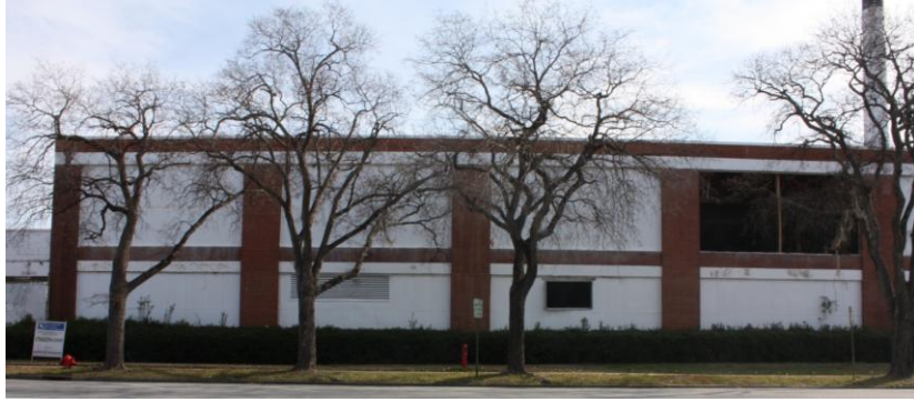
Figure 12: Photographer facing east, Photograph of Swift Mill’s weave shed added in 1945. Columbus, Muscogee County, Georgia, Photograph in possession of author, taken January 27, 2011. This addition, built with a steel frame, is similar to many International Style buildings, and even though it is multi storied, it looks very different from the older portions of Swift Mill.
