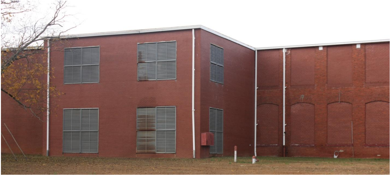
Figure 14: Photograph of Dunson Mill in LaGrange, Georgia. Photographer facing north, LaGrange, Troup County, Georgia, Photograph in possession of author taken November 16, 2010. Photograph of air washing and cooling tower. Cooling tower is in left center of photograph, to right of the conditioning tower is the original mill façade with bricked in windows.
