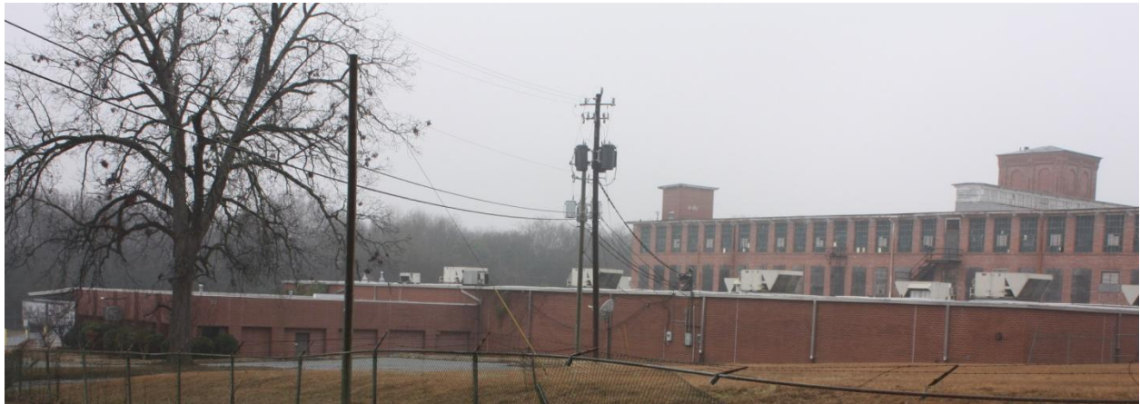
Figure 20: Photographer facing west, Photograph of one-storied addition at Macon’s Willingham Cotton Mills. Macon, Bibb County, Georgia, Photograph in possession of author taken February 1, 2011.
