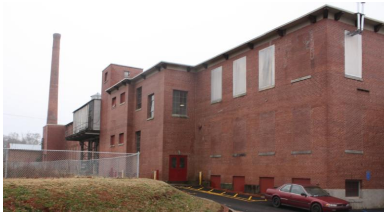
Figure 11: Photographer facing southwest, Photograph of Monroe Mill's 1949 addition. Monroe, Walton County, Georgia, Photograph in possession of author, taken January 18, 2011. The addition was built to fill in space between the main mill and areas where weaving was done. The addition is multi-storied, with window bays much like the original mill. The addition has been covered with an elevator shaft, toilet tower, and an air cleaning unit.
