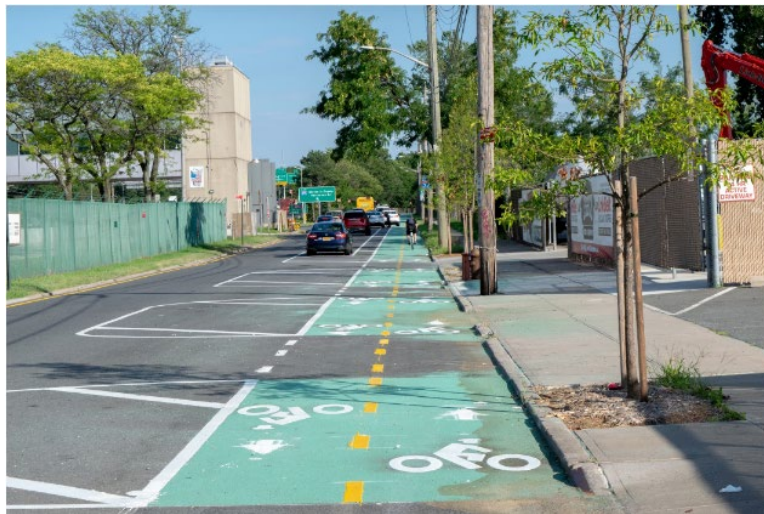
Retrofitting side streets with bicycle amenities can be done by marking new bike lanes with bright green paint and separating them from motor traffic by a series of bollards or a row of parked cars.
