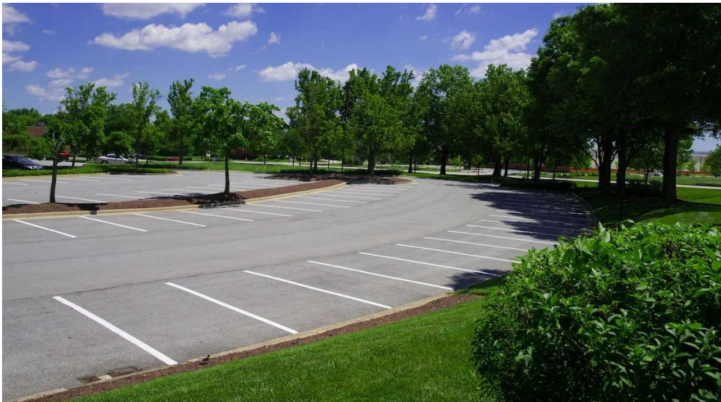
Planting landscaped tree islands in paved parking areas provides shade and mitigates any heat island effect.
