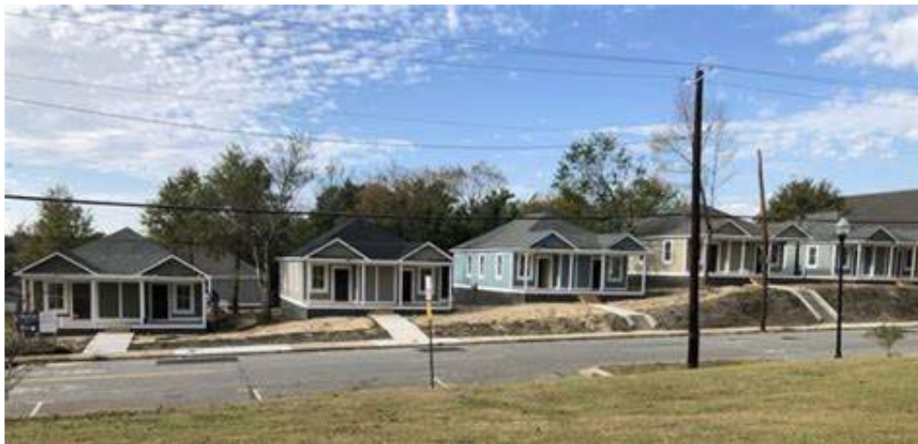
Newly constructed homes in the historic Beall's Hill neighborhood of Macon, GA. Historic Macon Foundation partnered with Mercer University, the Macon Housing Authority, and the John S. and James L. Knight Foundation to stabilize the neighborhood. Using historic architectural features such as gable roofs and front porches help new construction fit in existing neighborhoods while providing housing options at affordable prices.
