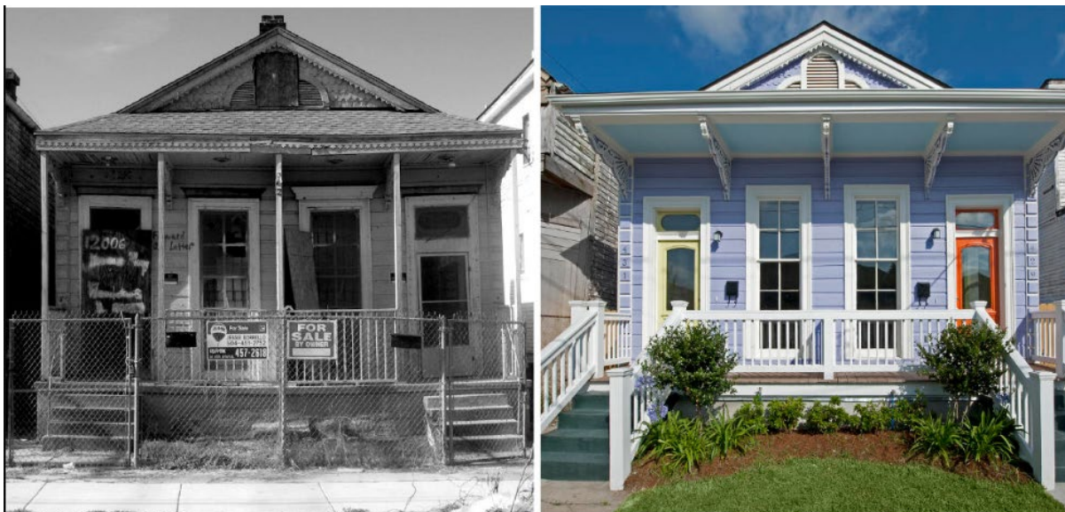
Example of rehab of historic duplex.
