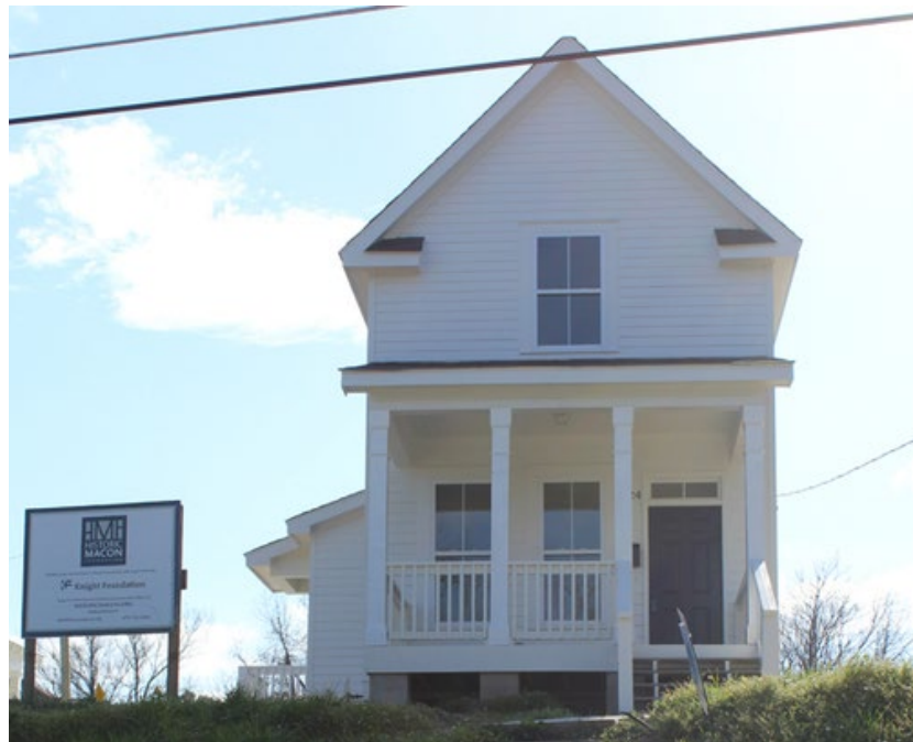
Newly constructed home at 932 Ash Street. Part of Historic Macon's Beall's Hill neighborhood stabilization project.
