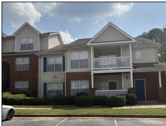
Existing building in eastern portion of the site
