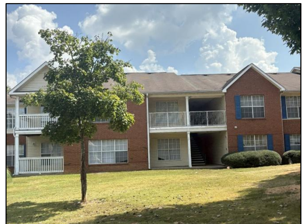
Existing building in western portion of the site
