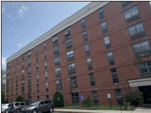
Subject property facing east
