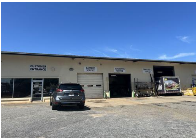
Commercial uses in the Subject's neighborhood
