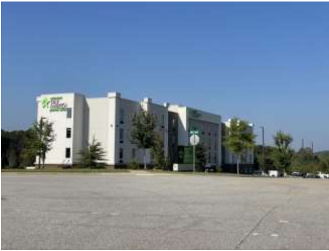
Hotel west of Subject site
