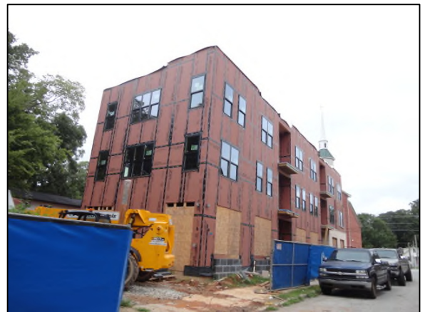
557 Lindsay Street Apartments (under construction) to the west
