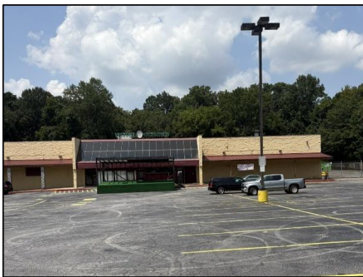
Existing building on site looking west
