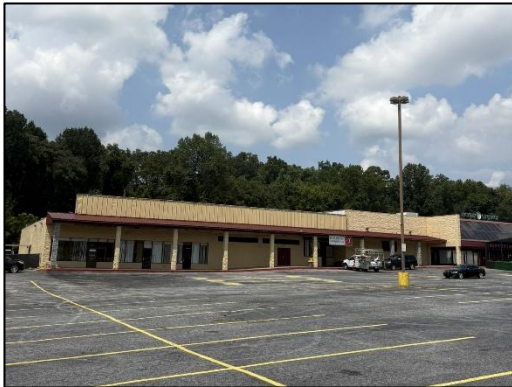
Existing building on site looking northwest
