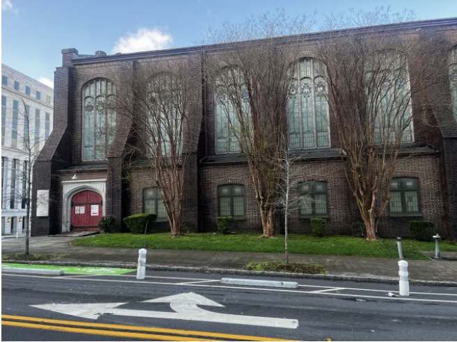
View of existing improvements on Subject site
