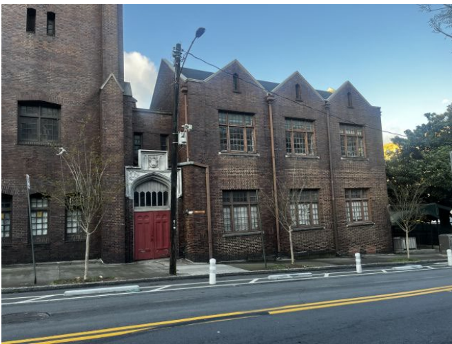
View of existing improvements on Subject site
