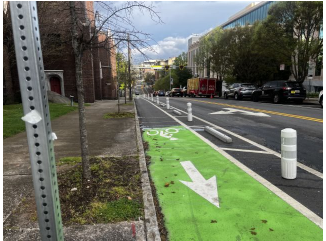
View of Trinity Avenue SW facing northwest
