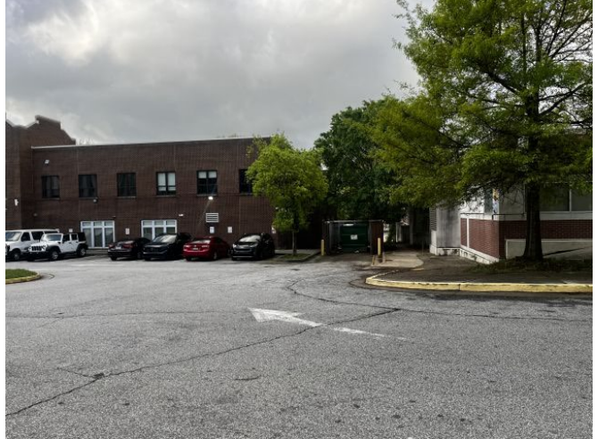
Parking garage immediately southwest of Subject site
