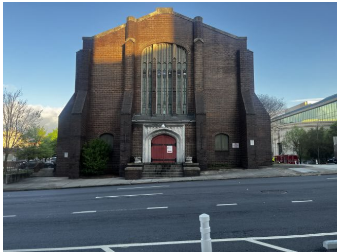
View of existing improvements on Subject site
