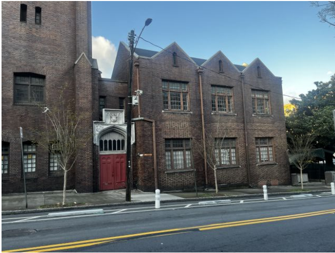
View of existing improvements on Subject site
