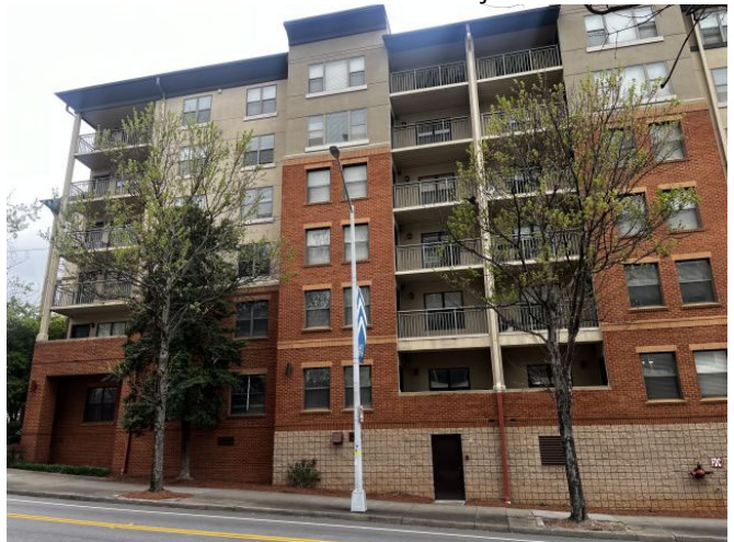
City Plaza (comparable property) northwest of Subject site
