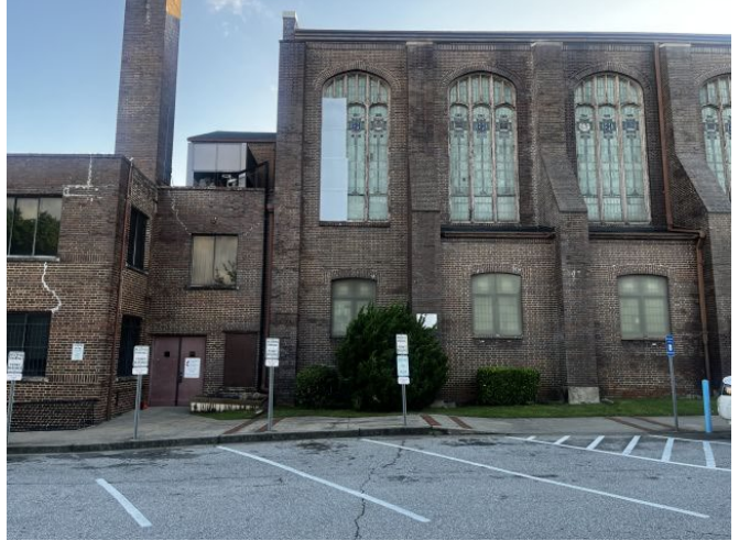
View of existing improvements on Subject site
