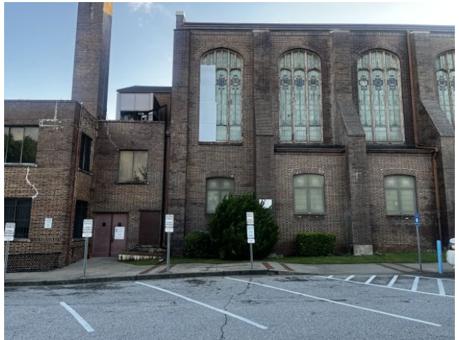
View of existing improvements on Subject site
