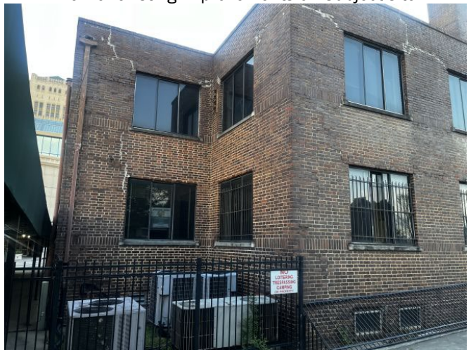
View of existing improvements on Subject site
