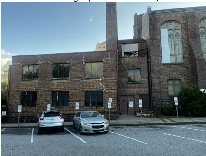
View of existing improvements on Subject site
