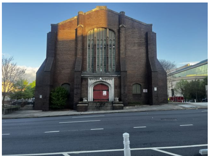
View of existing improvements on Subject site
