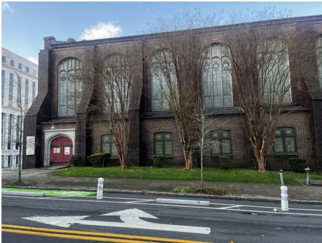
View of existing improvements on Subject site
