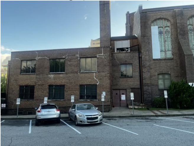
View of existing improvements on Subject site
