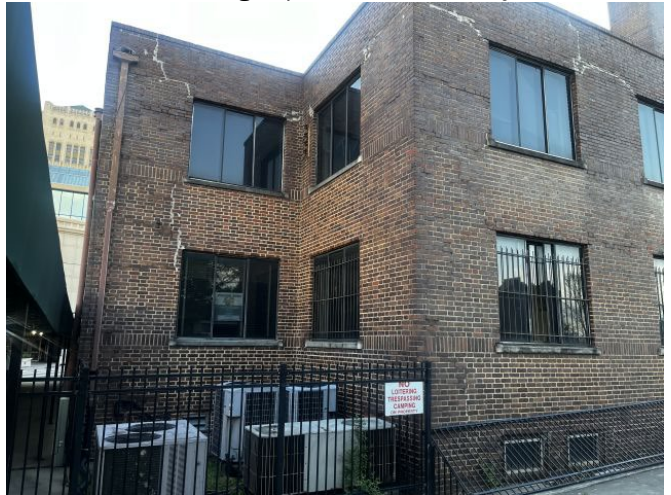
View of existing improvements on Subject site
