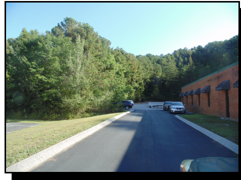
(4) Site off US 27, west to east.
