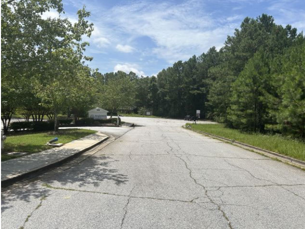
View along Manchester Drive facing south
