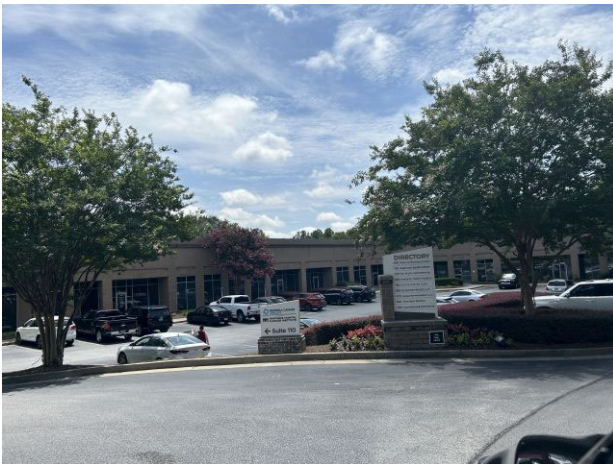
Medical office building to the east
