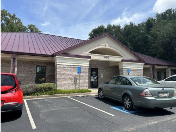
Medical office building to the east
