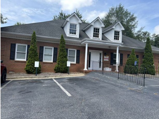
Medical office building to the east
