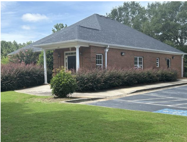
Medical office building to the east
