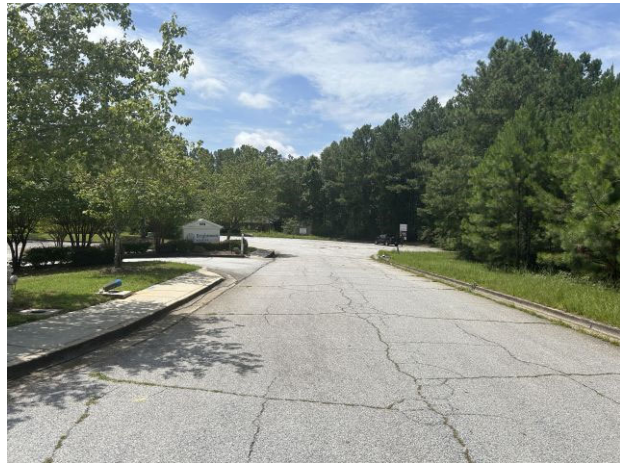
View along Manchester Drive facing south
