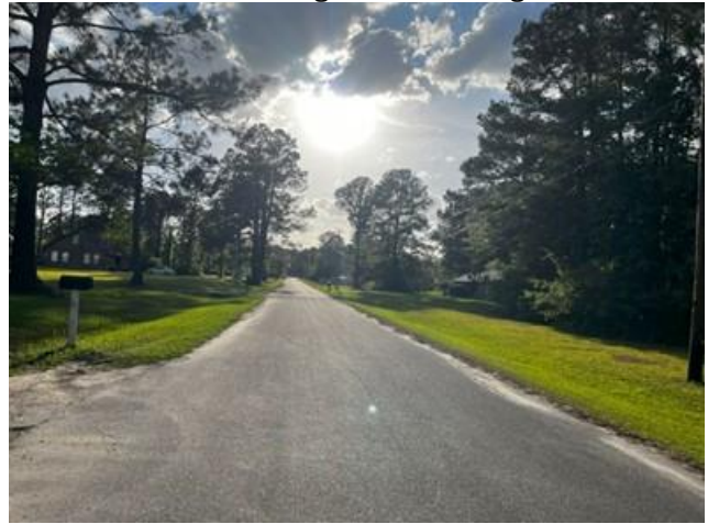
View of Windsor Avenue facing west
