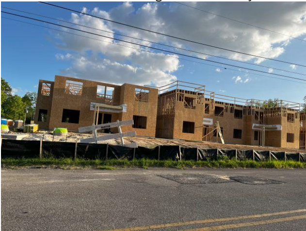
Dogwood Trace under construction
