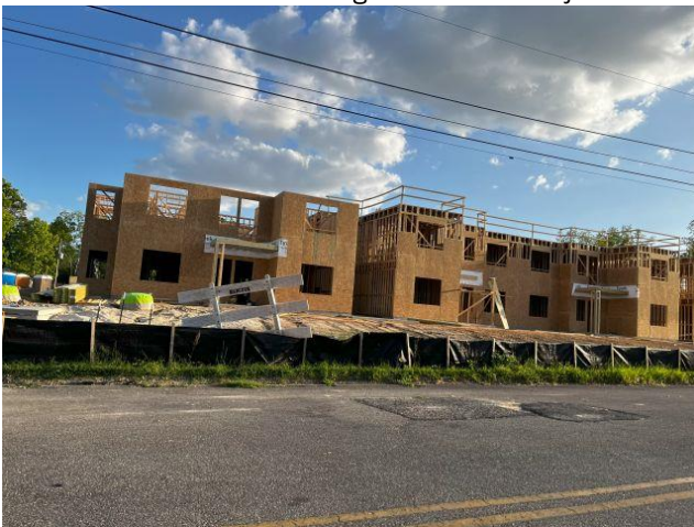
Dogwood Trace under construction
