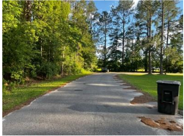
View of Greenridge Avenue facing south
