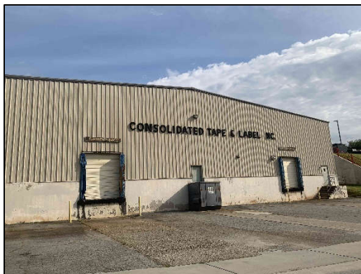
Consolidated Tape and Label Co. bordering the site to the west
