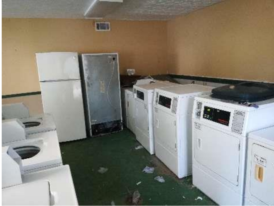
View of Laundry Facility
