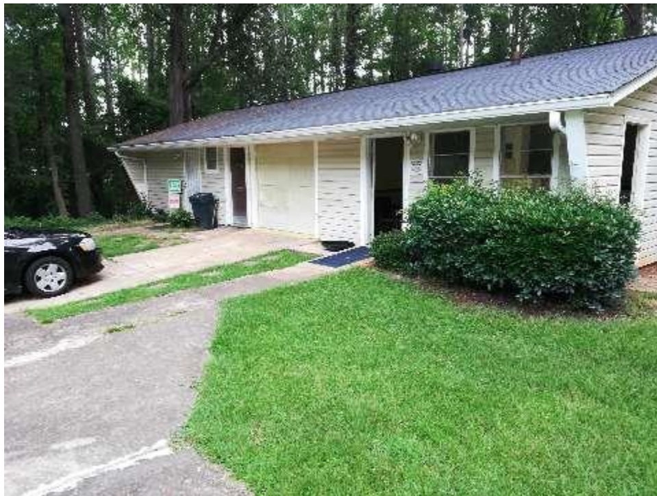
View of Accessory Building - Exterior
