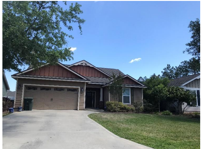
Single-family homes west of the Subject site
