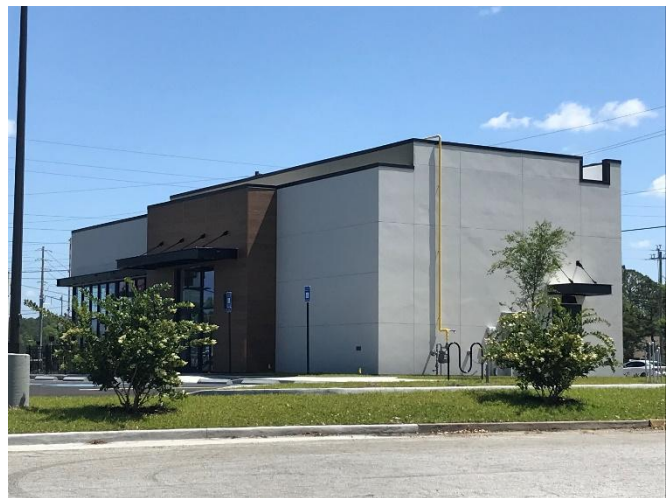
Under construction Starbucks north of the Subject site
