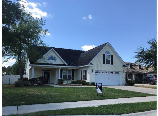
Single-family homes west of the Subject site
