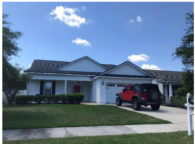
Single-family homes west of the Subject site
