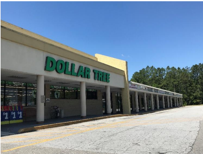
Commercial plaza northwest of the Subject site on E King Avenue
