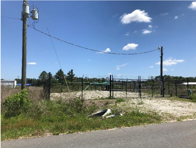
Utilities northeast of the Subject site
