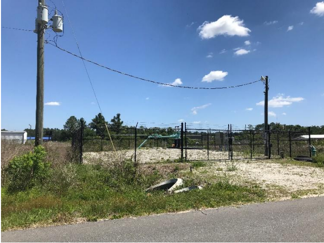
Utilities northeast of the Subject site
