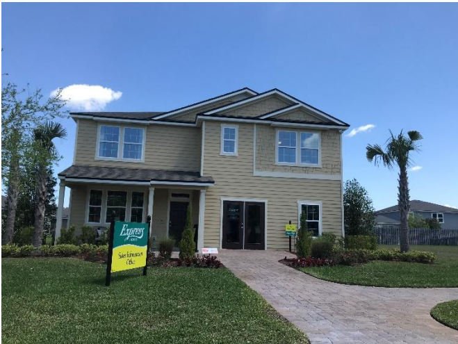
Single-family homes west of the Subject site
