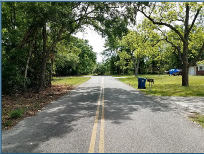
Streetscape: East View of West 3rd Street
