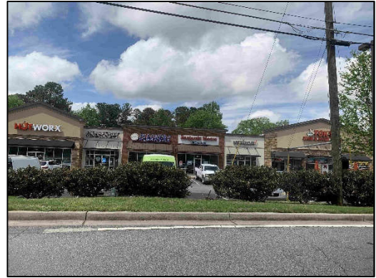
A retail shopping center just northeast of the subject site
