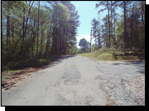
(3) From site entrance north along Emmanuel Harris Rd.
