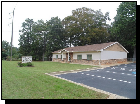
(11) Animal Hospital, across from site off SR 113.
