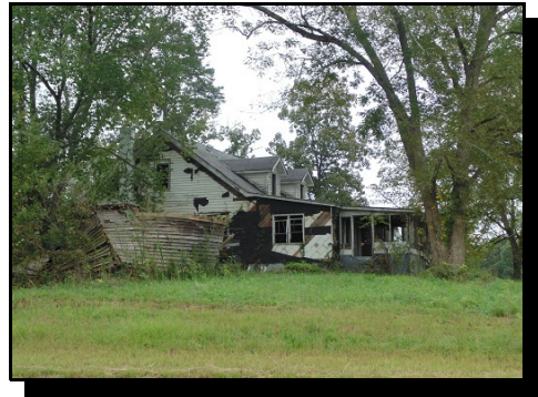
(8) House on site that will be demolished.
