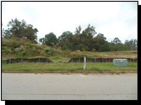
(5) Site off Northwinds Blvd, North to south.
