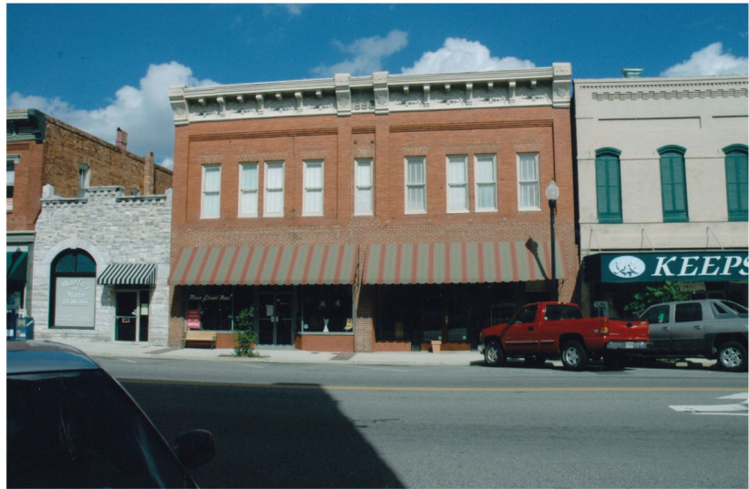
The Tifton Commercial Historic District was enhanced by the rehabilitation of this circa 1896 commercial building for $222,606 in private investment.
