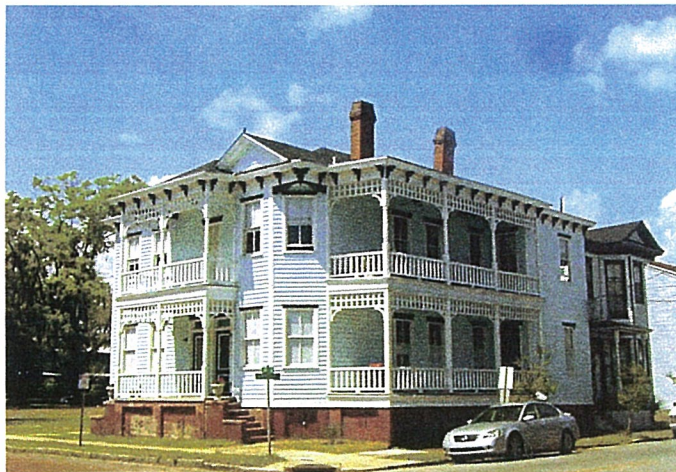
Duplex rehabilitation in Savannah representing $180,000 in private investment.
