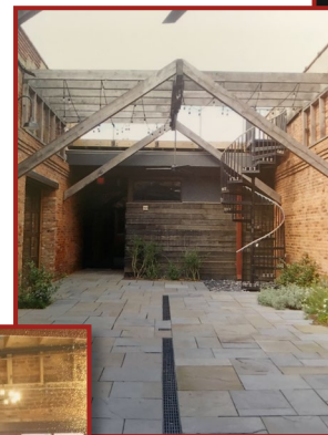
The center bay's roof had collapsed before the building was purchased by the current owner. This circumstance gave them the flexibility to leave the area open and just repair the remaining roof structure. Other work included structural repair and stabilization and repair to the building materials.
