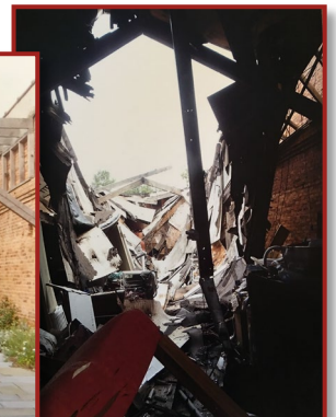
The center bay's roof had collapsed before the building was purchased by the current owner. This circumstance gave them the flexibility to leave the area open and just repair the remaining roof structure. Other work included structural repair and stabilization and repair to the building materials.
