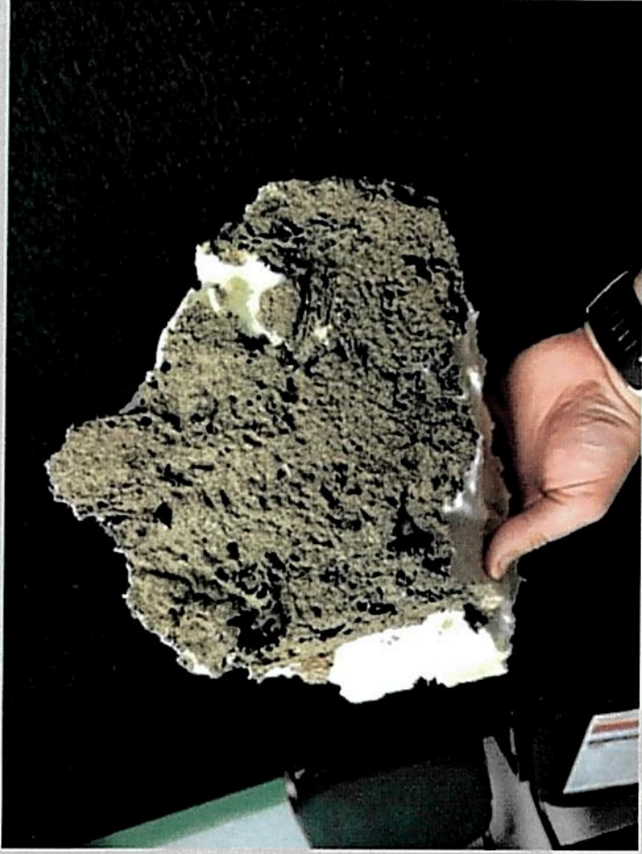
Back side of of spray foam
