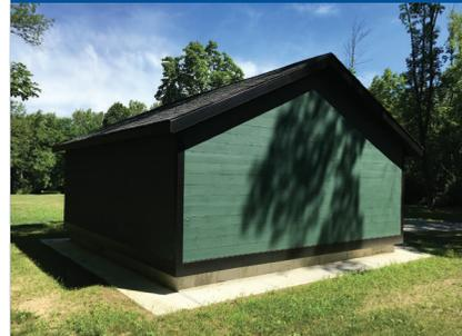
PHOTO 4 Concrete skirt perimeter pest-resistant ground break.
