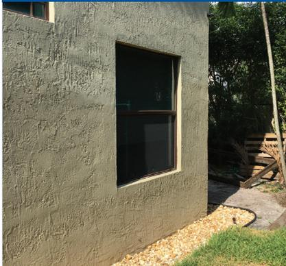
PHOTO 2 Pea gravel-crushed stone perimeter pest-resistant ground break.
