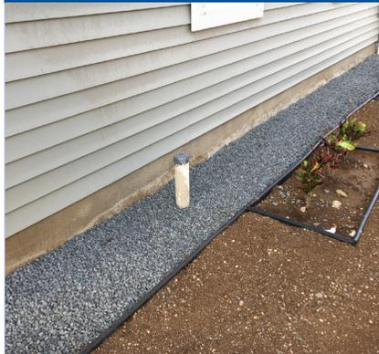
PHOTO 3 Concrete skirt perimeter pest-resistant ground break.
