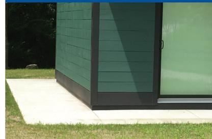
PHOTO 5 Concrete paver perimeter pest-resistant ground break. (Photo courtesy of the San Francisco Department of the Environment—Pest Prevention by Design.)
