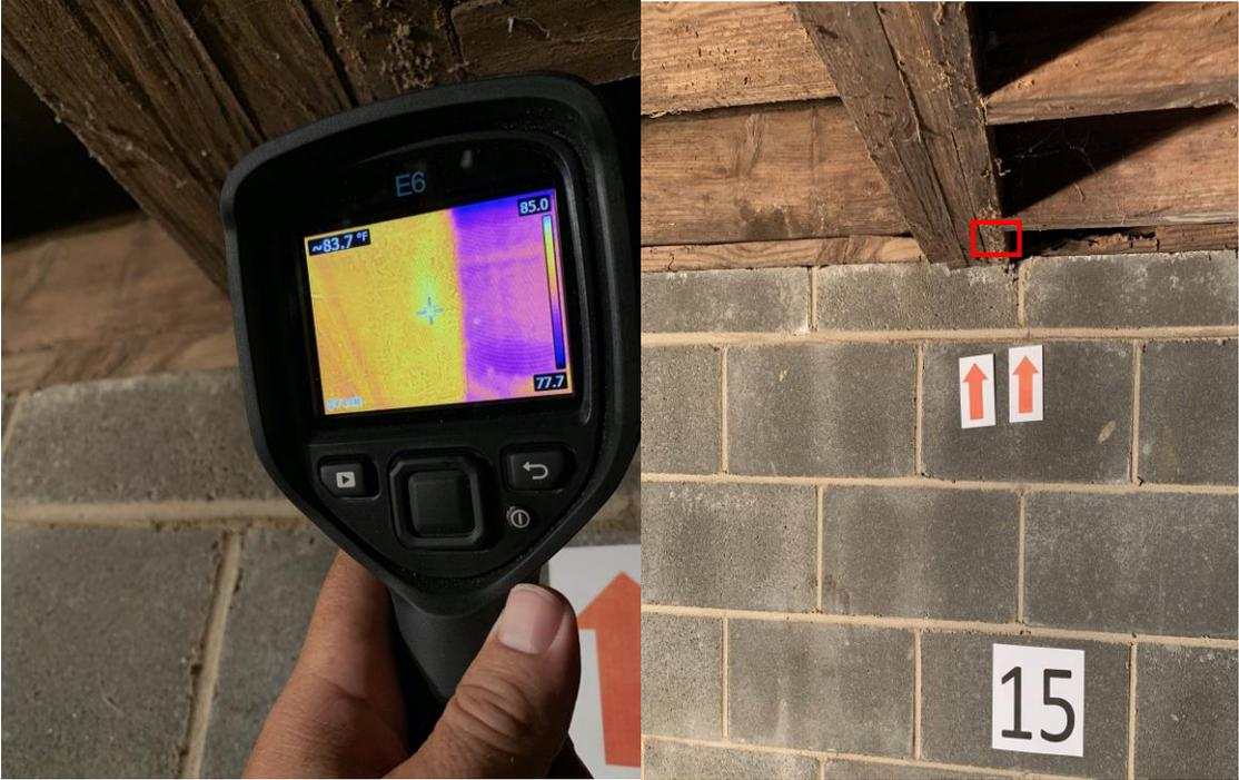
Photograph 3. Images of termite activity in the SPF observed during the August inspection from the joists and joist header by Location 5.
