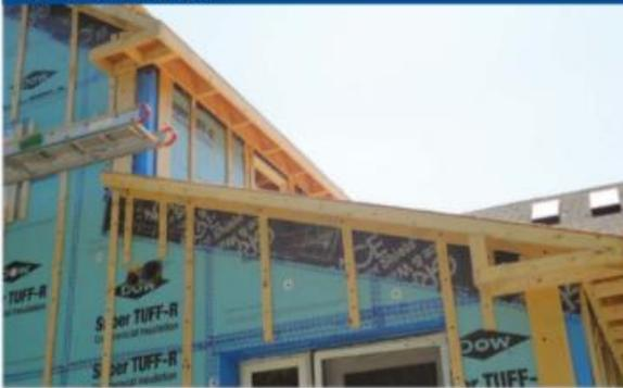
PHOTO 2 Extruded Polystyrene (XPS) Boards. The rigid insulation boards are installed on the exterior of framing with their joints taped/sealed and act as the water control layer, air control layer, vapor control layer and thermal control layer—all four control layers.
