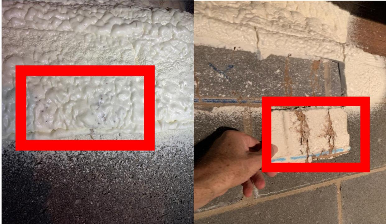
Photograph 5. Images from the borescope showing SPF without (left) and with (right) termite activity.
