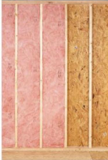
PHOTO 11 Faced Insulation Batts. Airflow and convection can be effectively controlled by facers adhered to batt insulation. Note that faced insulation batts should have the facers installed to the face of the stud framing, not inset stapled. Inset stapling creates voids and air channels that can lead to convective loops and a loss of thermal resistance.
