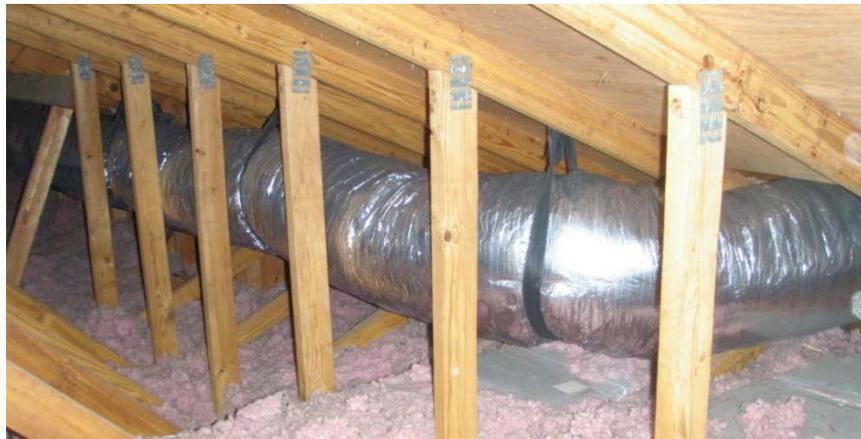
**Figure 9. Return ductwork for House 2**
