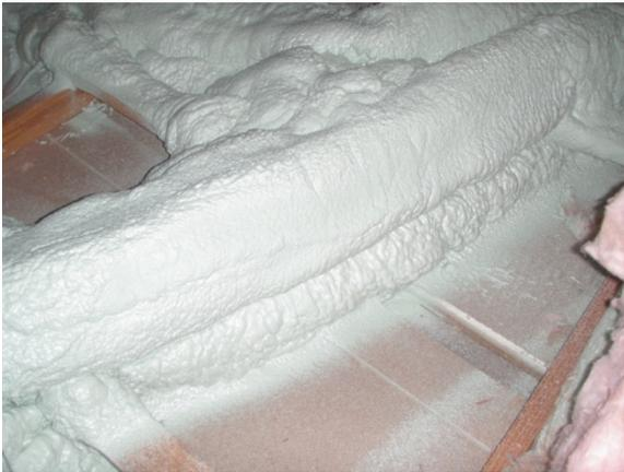
**Figure 20. Ductwork well-sealed to sheetrock with ccSPF**
