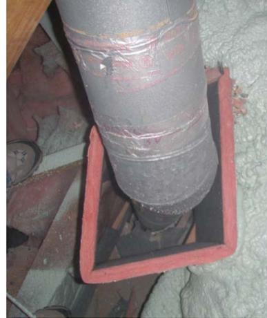
6. Encapsulate ductwork in at least 1.5 in. of ccSPF. The minimum thickness must be maintained consistently on all sides to mitigate condensation concerns.
