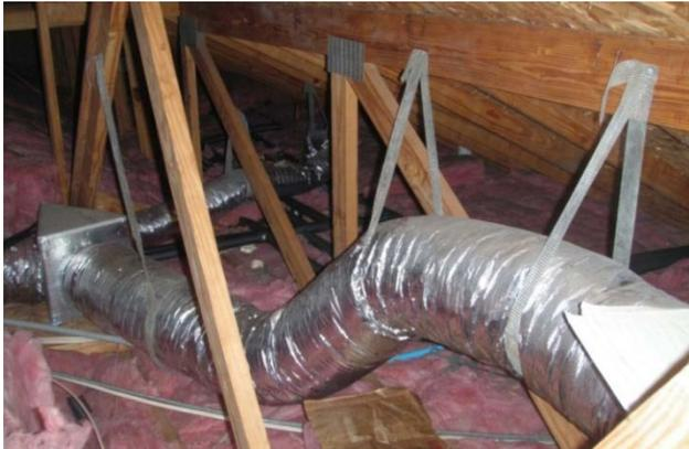
**Figure 1. Traditional ductwork hung from attic rafters**
