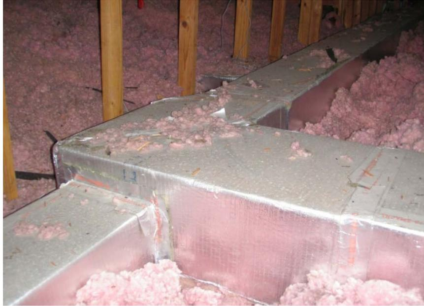
**Figure 8. Supply ductwork for House 2**
