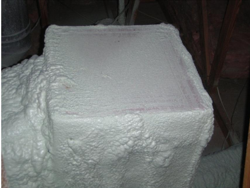
**Figure 17. Improperly spray-foamed plenum box at House 1**
