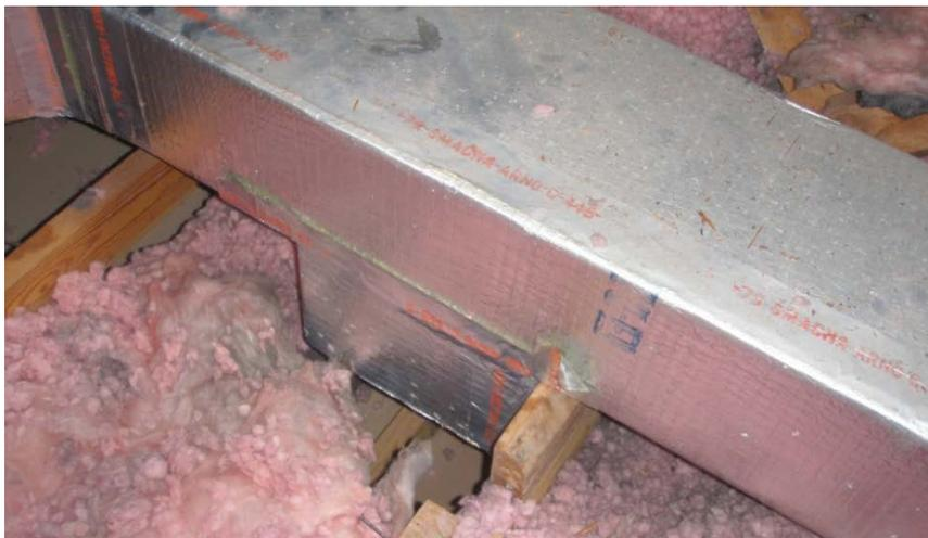
**Figure 12. Open duct take-off at House 2**
