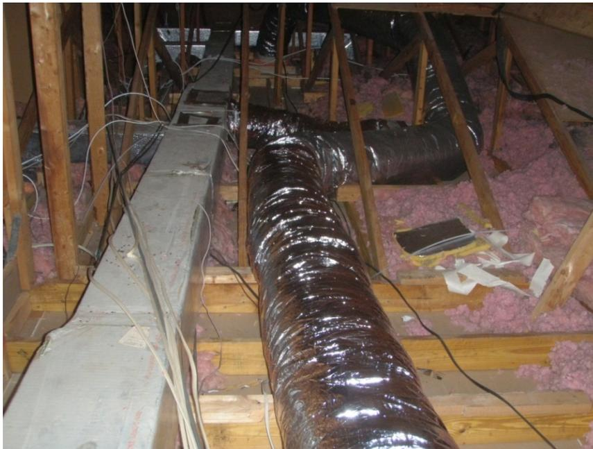
**Figure 11. Duct reconfiguration at House 2**
