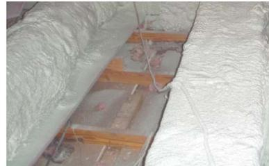
7. Bury encapsulated ductwork in loose-fill insulation. The insulation must cover the ductwork to be considered fully buried. Code requires a minimum of 1.5 in. of coverage over the ducts for ccSPF materials that do not meet the flame spread requirements. Coverage of 3.5 in. over the duct surface achieves a deeply buried rating.
