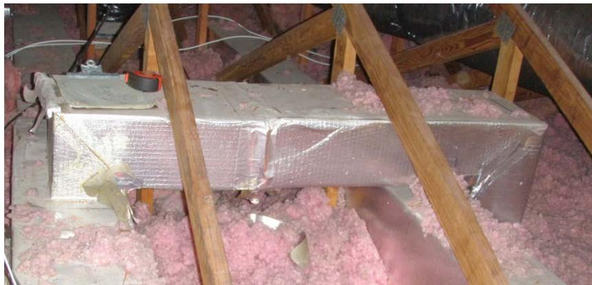
**Figure 10. Supply ductwork jump over abandoned return ductwork**
