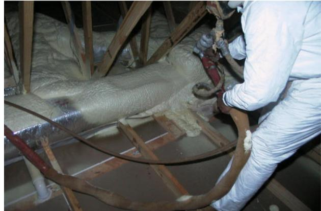
**Figure 2. Ducts being encapsulated with ccSPF**
