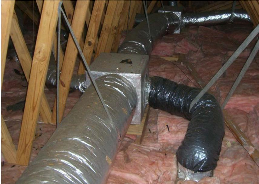
**Figure 7. Existing ductwork at House 1**
