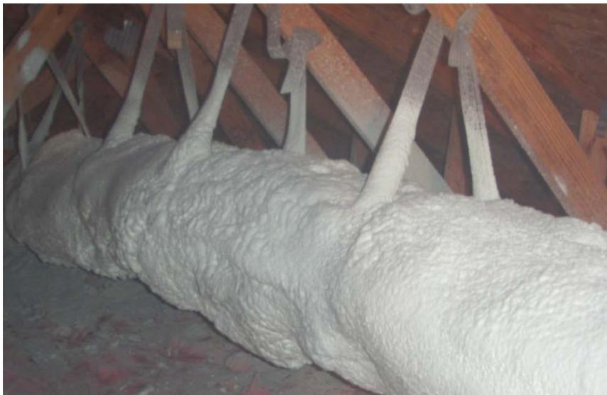
**Figure 13. Finished encapsulated duct hung from roof deck**
