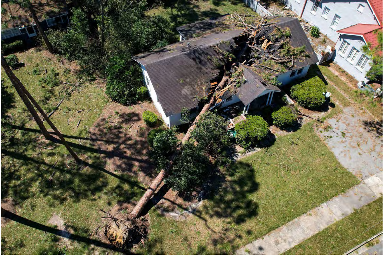
Figure 1: Photo: Hurricane Helene Damage (Source: John Falchetto / The Atlantic, 09/25/24)
